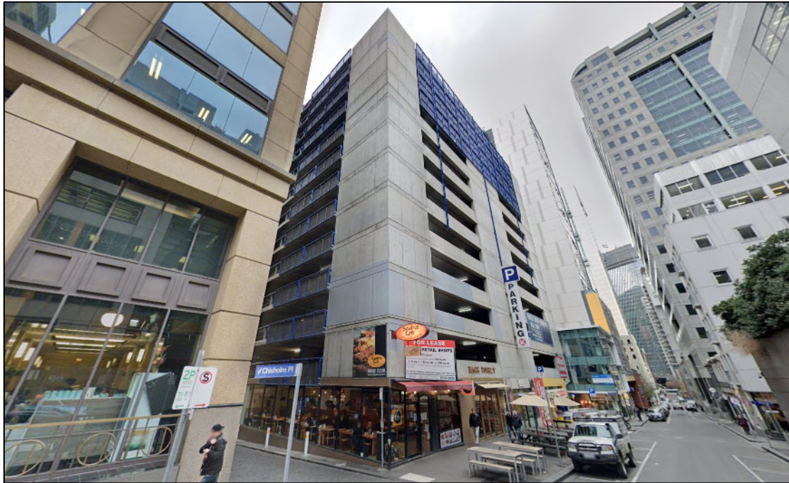
Figure 3 – The site, street view (Little Lonsdale Street)
