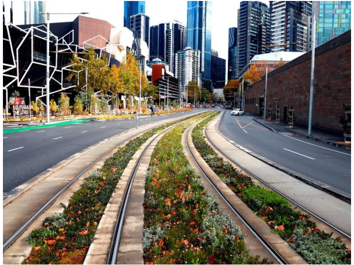
Stage 1 roadway and tram works - complete
