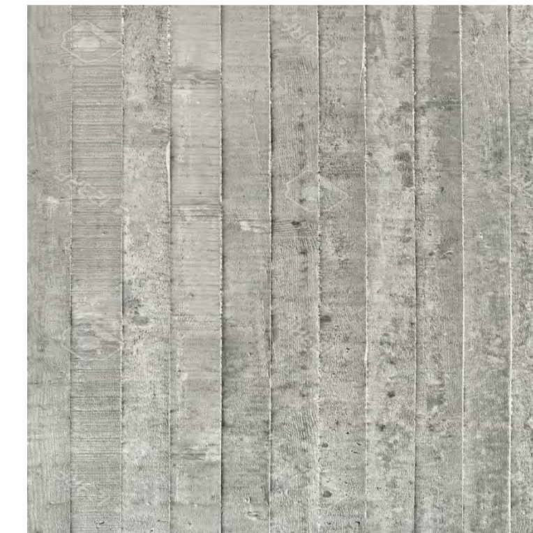
CN05 - BOARD FORMED PRECAST CONCRETE
