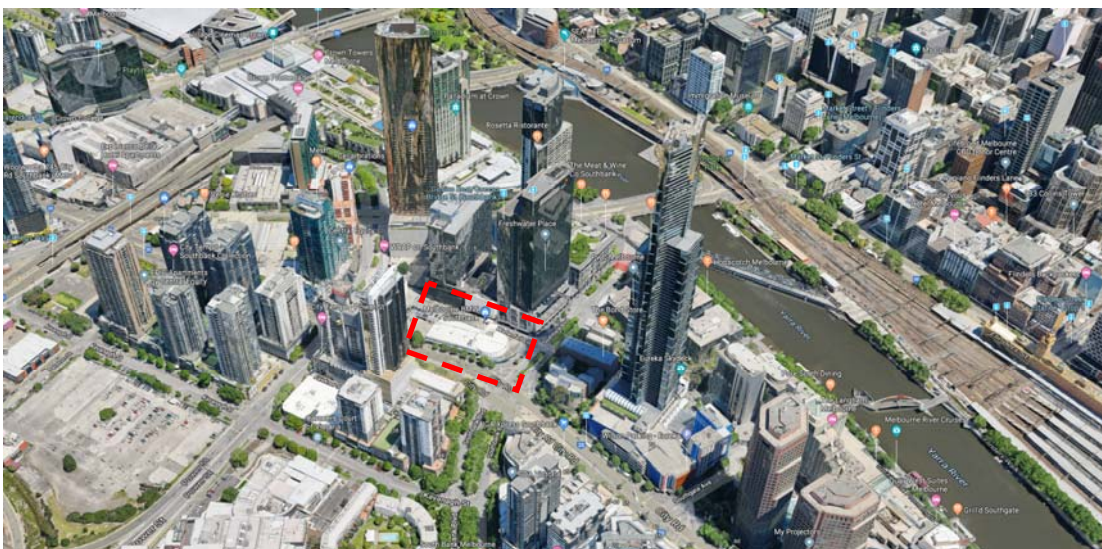
Figure 4: 3D aerial of subject site's immediate built form context (Google Maps)
