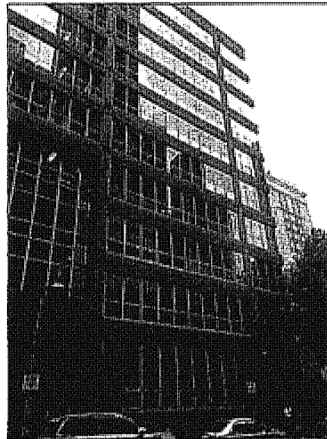
Figure A.6. 661 Bourke Street – Little Collins Street elevation
