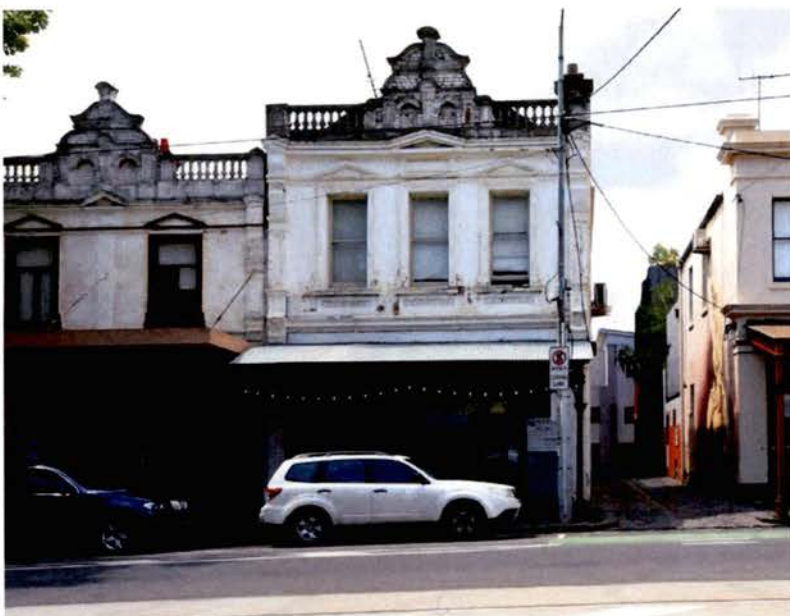
Figure 7 550 Queensbury Street before and after awning reconstruction.
