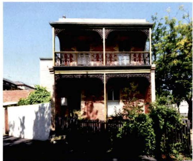
Figure 9 Morrah Street, Parkville - before and after paint removal
