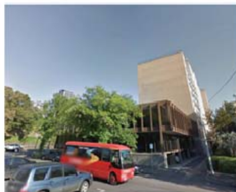
VIEW 2 Looking towards subject site along Batman St.
