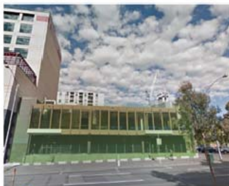
VIEW 1 Looking towards subject site from the edge of Flagstaff Gardens.
