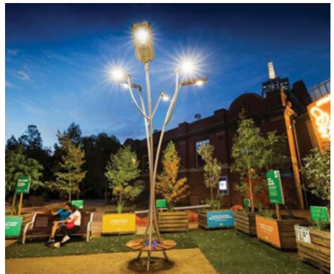
Image 8: 'Solar tree' (Birraring Marr, 2018) is an award-winning example of innovation developed by City of Melbourne's own designers. The tree captures solar energy to charge LED lighting and USB sockets.
