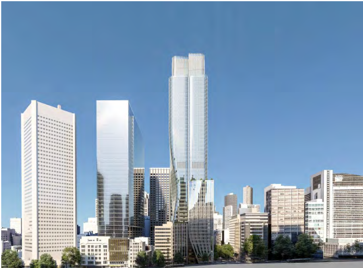
Perspective from Bourke Street (north elevation) of the proposal and surrounds (Bate Smart September 2019)
