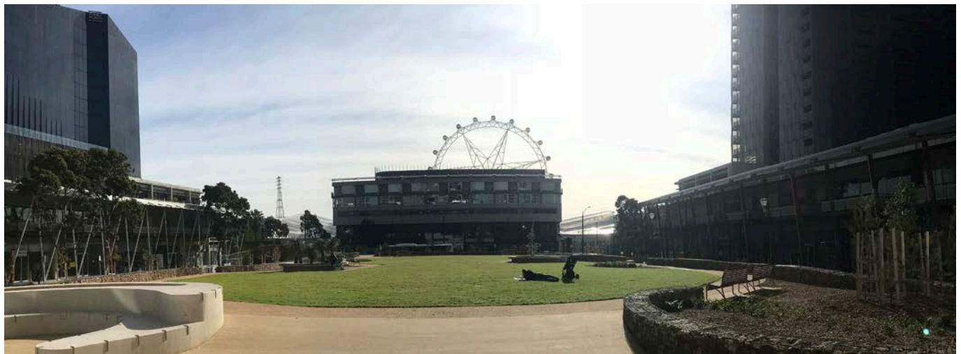
Figure 2. DD - View from NewQuay Central Park towards the Development Sites (air rights)
