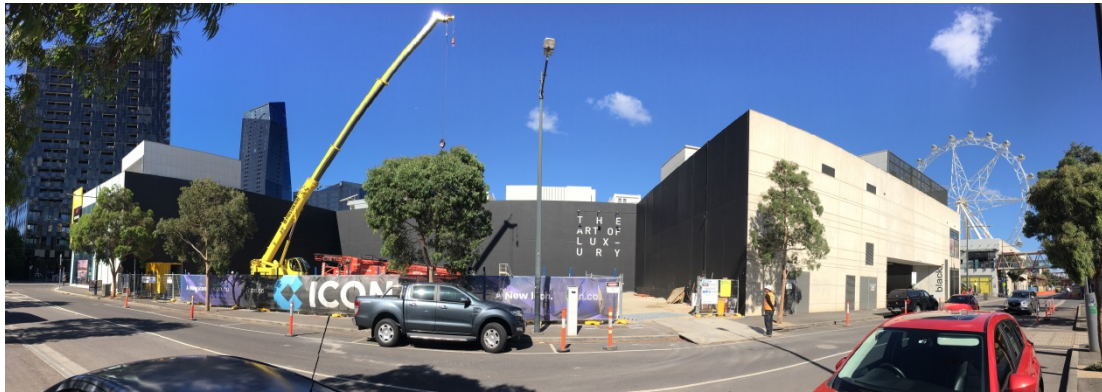
Figure 5 - View of SE Site from Waterfront Way
