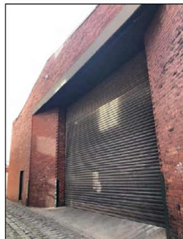
Figure 2: Pinkys Lane Photograph of Subject Site
