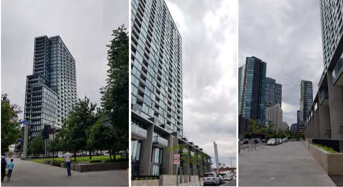
Views: 1. south west over Buluk Park; 2 south west along Collins St; 3 east along Collins St January 2019 photos of CW1 - 915-941 Collins St Docklands
