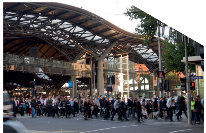
Crossing Spencer Street at Southern Cross Station
