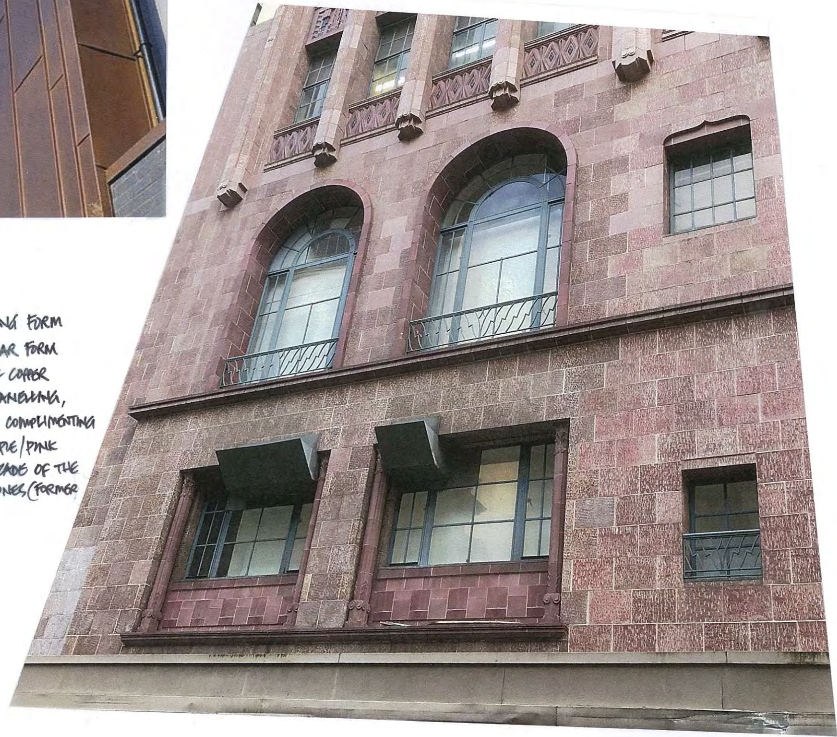
LT. COLLINS STREET DAVID JONES STORE (FORMER COLES BUILDING) FACADE
