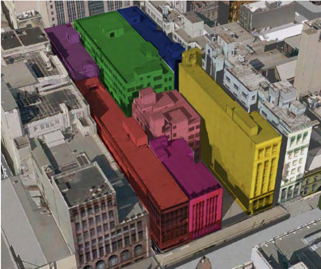
Figure 3: Collection of 8 buildings (note building internal to the site)
