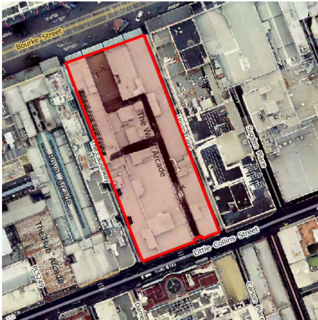
Figure 2: Aerial photograph. Note the Arco building internal to the site.
