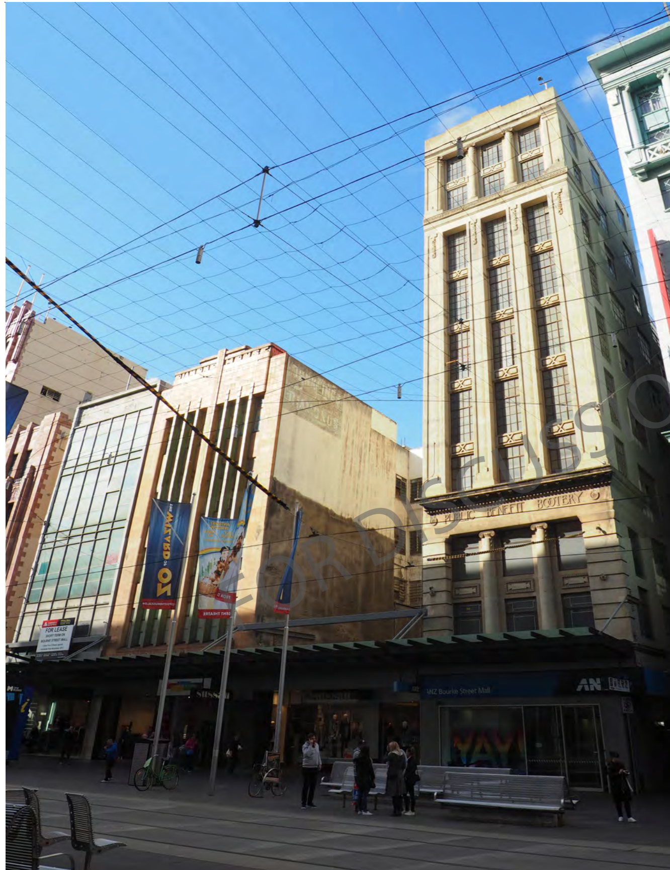
EXISTING BUILDING FACADE
