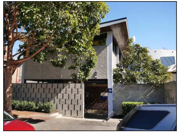
Source: Applicant's site photo, April 2018
