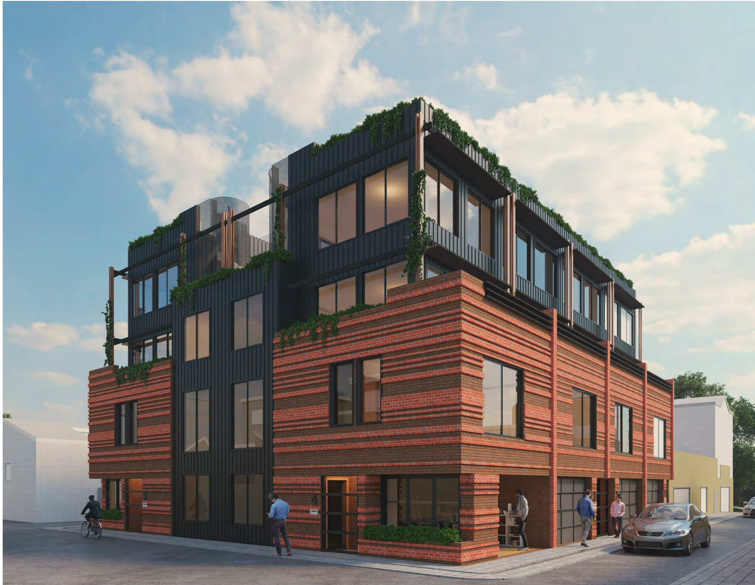
EARLIER REVISION RENDER - RENDER TO BE UPDATED TO REFLECT THE CURRENT DESIGN
