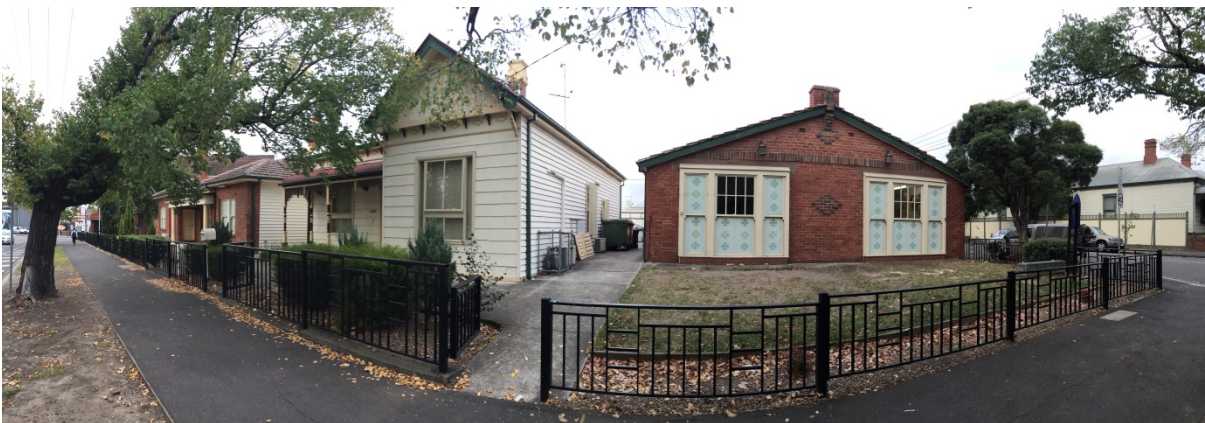
Figure 6: Subject site (7 & 9-11 Epsom Road)
