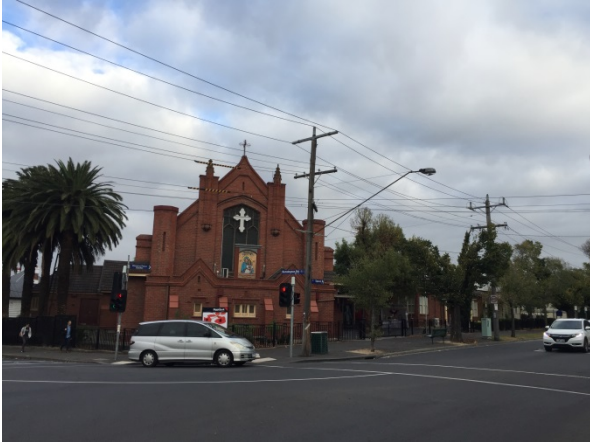
Figure 3: Subject site (1-3 Epsom Road)
