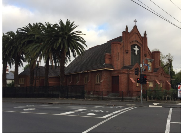
Figure 4: Subject site (1-3 Epsom Road)
