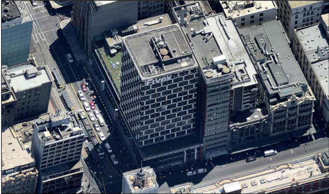
Figure 2 - Existing South Facing High-Wall Sign
