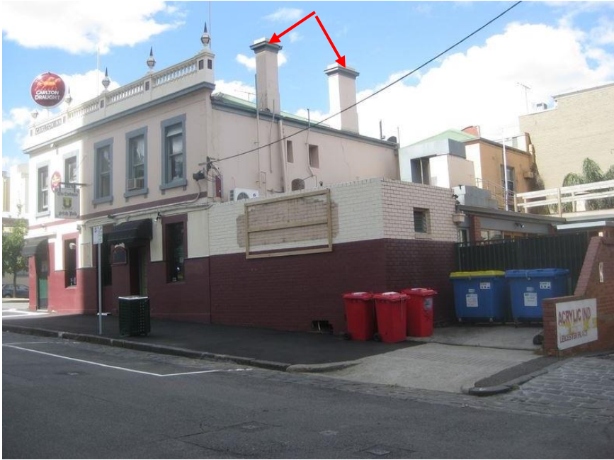
Carlton Inn, rear along Leicester Street, showing visibility of original chimneys (Source: City of Melbourne Interactive Map, circa 2015)
