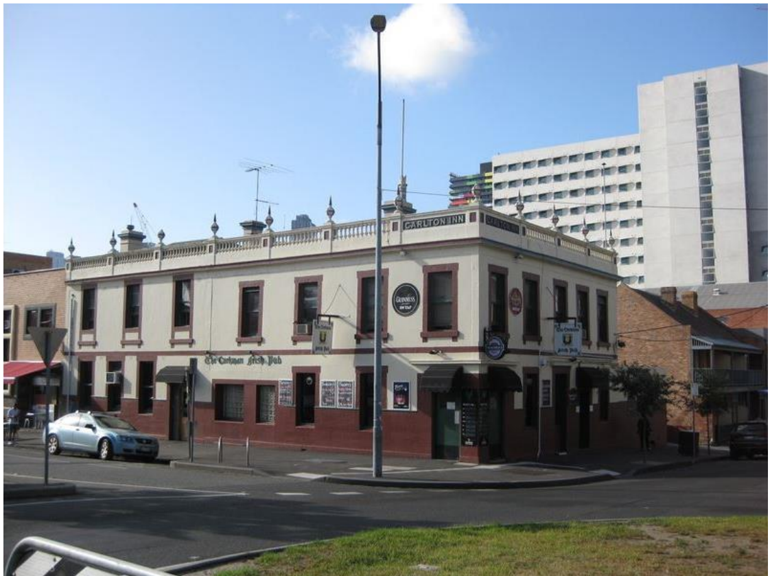
Corner of Pelham and Leicester streets, showing relationship to adjacent HOs to the Carlton Inn (Source: City of Melbourne Interactive Map, circa 2016)
