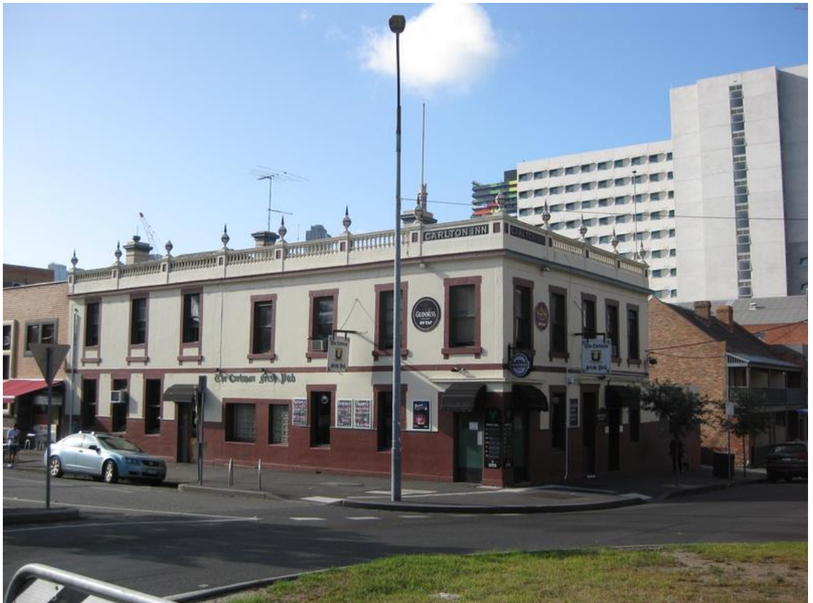
Figure 1 – Image of former Hotel building on site (Source: maps.melbourne.vic.gov.au )- pre-demolition.
