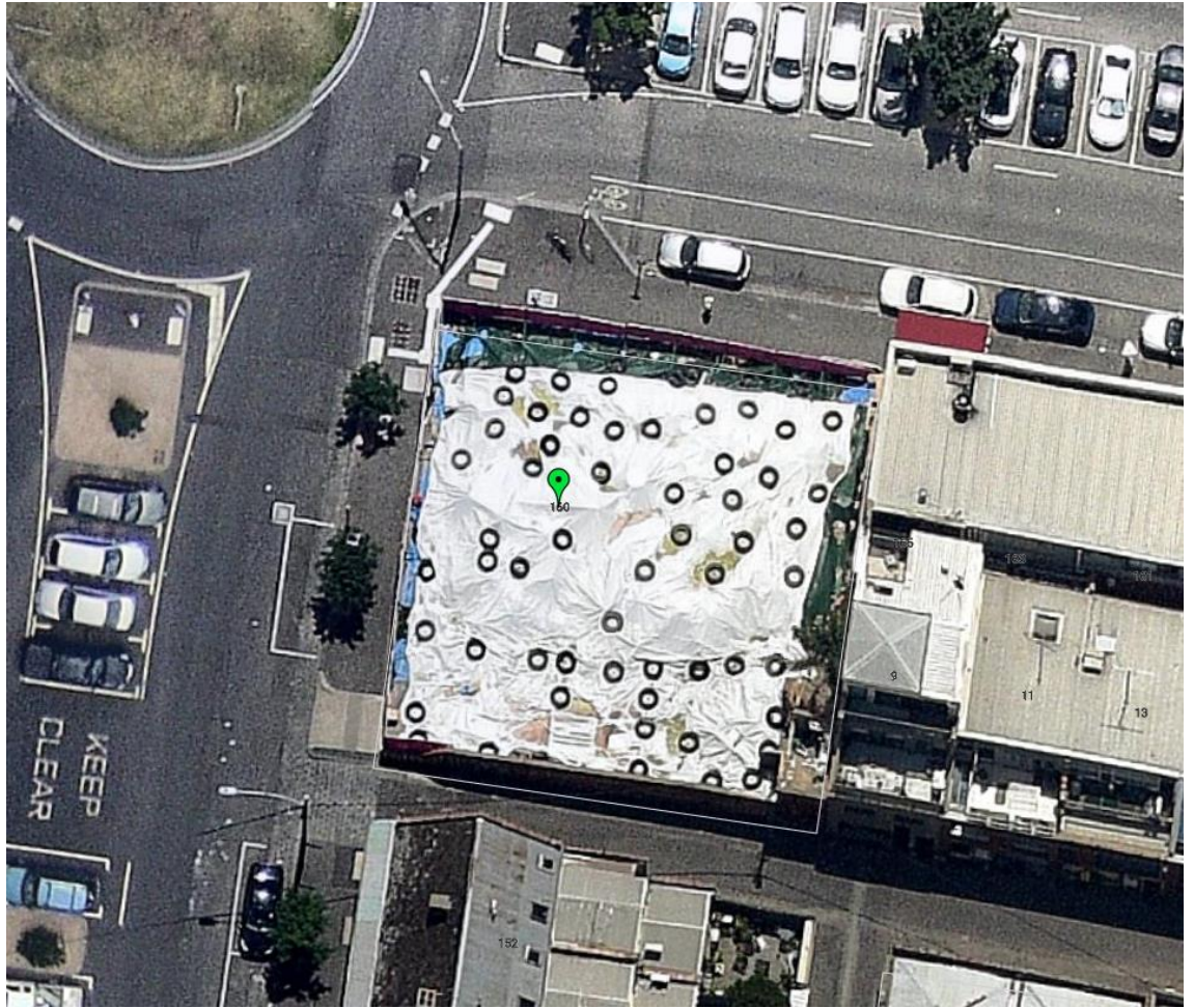
Figure 7 – Aerial Photo – 23 November 2017 (Source: Nearmap) – post demolition.
