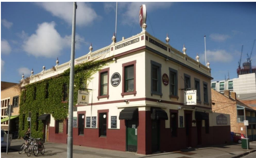
Carlton Inn, mid-2011 Comparison with the earlier photograph shows that it was largely intact to its earlier 20 th century appearance NB the tiled dado had been painted over (Source: RBA)
