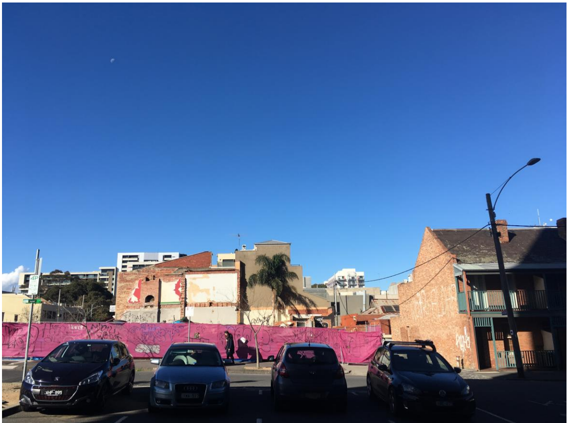
Figure 4 – View towards subject site looking across Leicester Street with four storey adjoining development in centre and two storey brick heritage properties to right (over Leicester Place).
