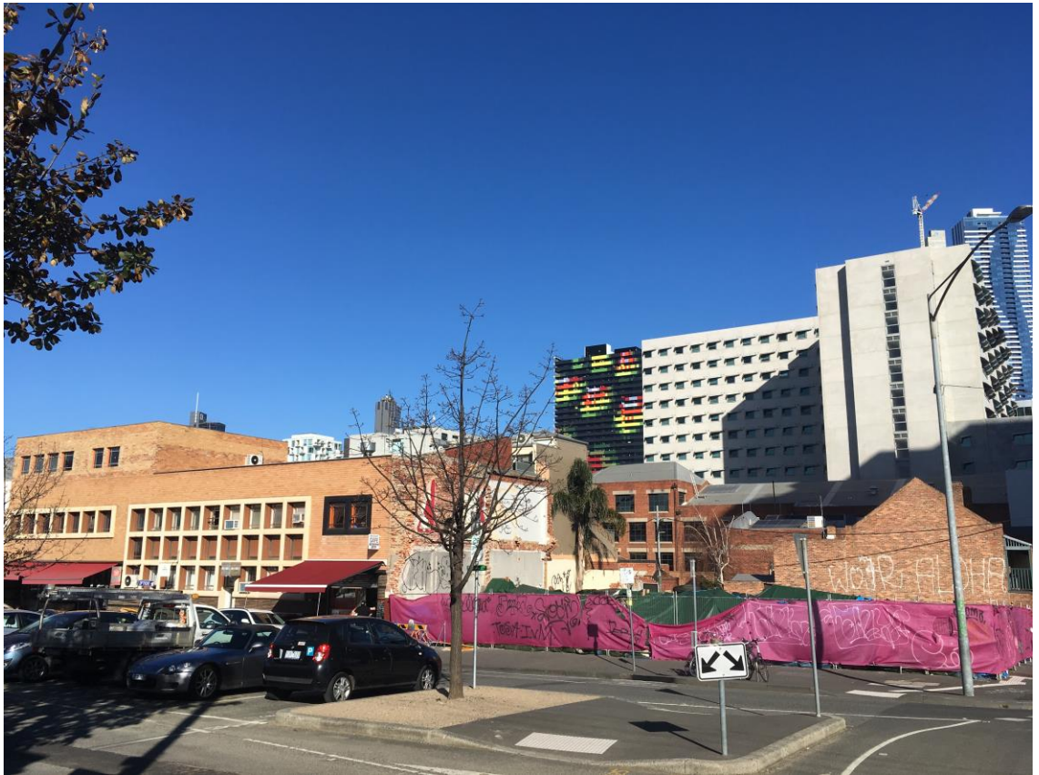
Figure 3 – View of site looking generally south across Pelham Street with two to three storey former warehouse building to left.
