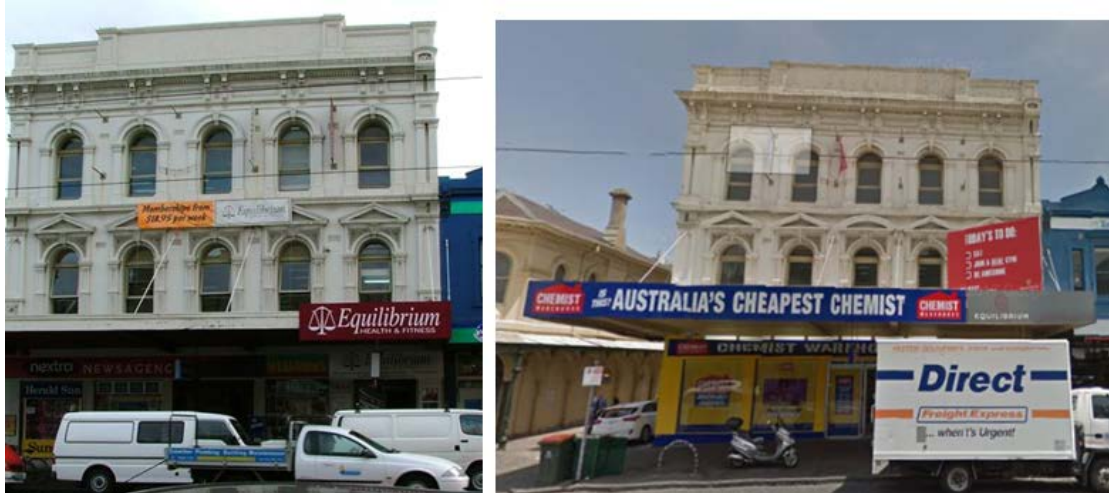
Image showing width of fascia before and after (the Equilibrium fascia sign does not have a permit)
