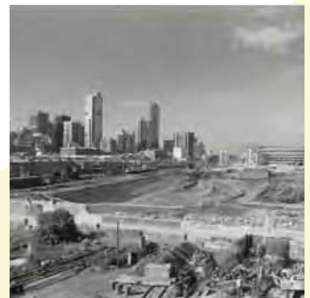
Looking south east showing the excavation of Docklands - 2000 Photographer: Ian Harrison Hill
