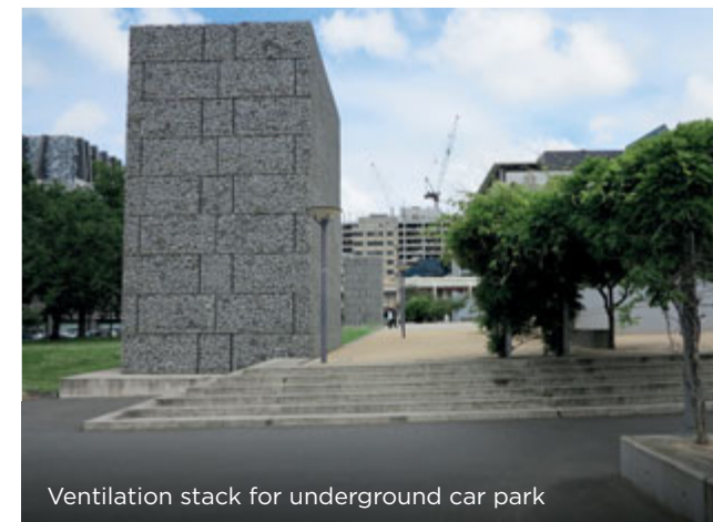
Plaza looking south towards Pelham Street
