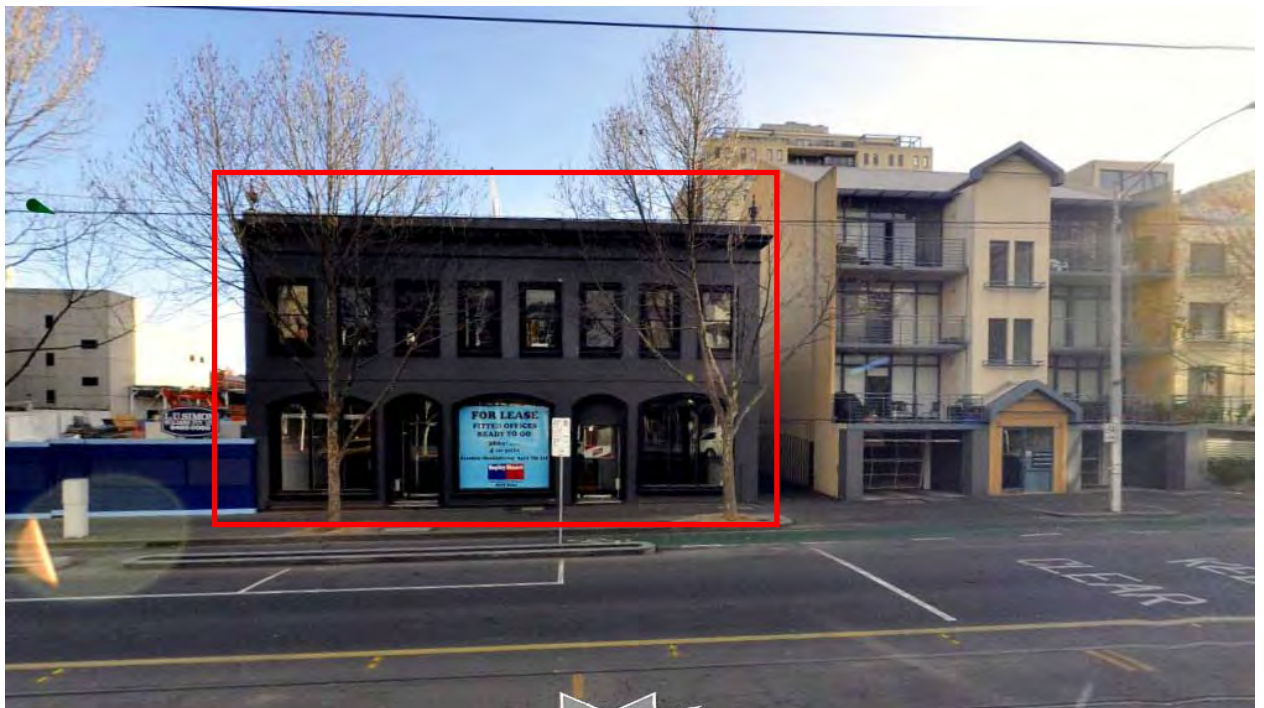
Figure 2: Photo of existing building on the subject site which is proposed to be demolished.
