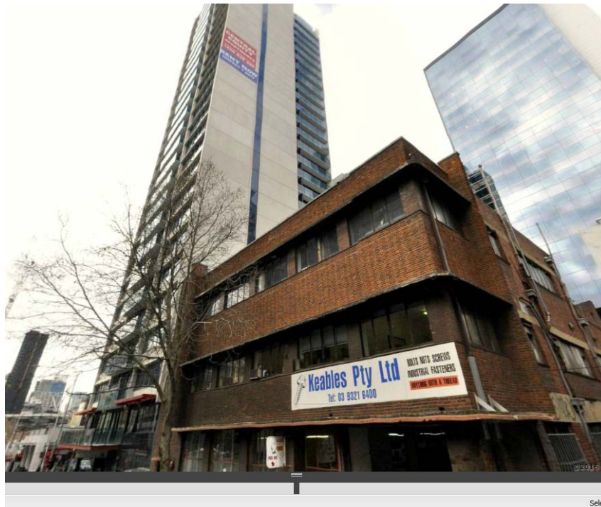
Figure 2: Streetscape view of the existing B graded building on the subject site and the adjoining 29 storey residential development located to the immediate east of the site at 175-181 A'Beckett Street.
