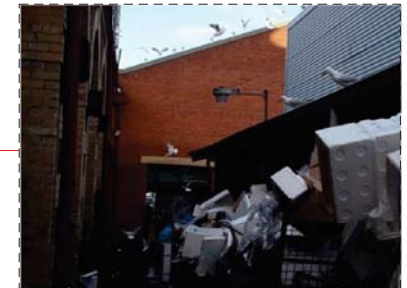
INADEQUATE SERVICE AREAS OPEN TO AIR
