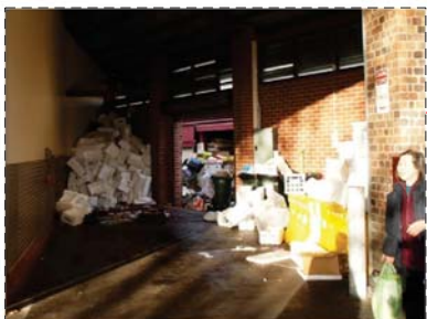
INADEQUATE WASTE TRANSFER FACILITIES
