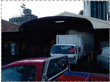
THE MEAT HALL LOADING DOCK IS INADEQUATE
