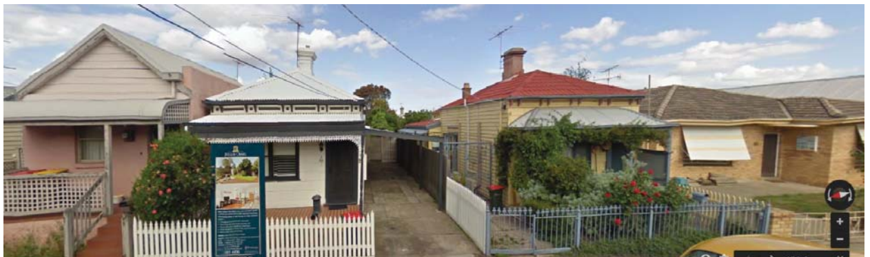
Figure 5. From left, 31, 33, 35 and 37 Barrett Street. Numbers 35 and 37 are proposed to be demolished.
