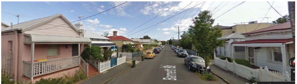
Figure 2. Barnett Street looking south. Red roof on left is number 35 proposed to be demolished (Google Streetview)
