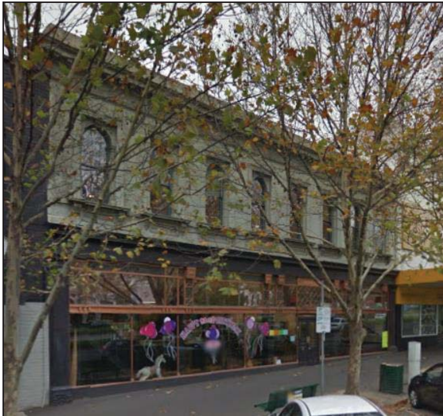
View of 535-541 Elizabeth Street – Source - Google Streetview June 2014).
