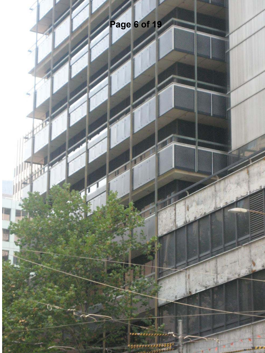
New cladding to William Street facade
