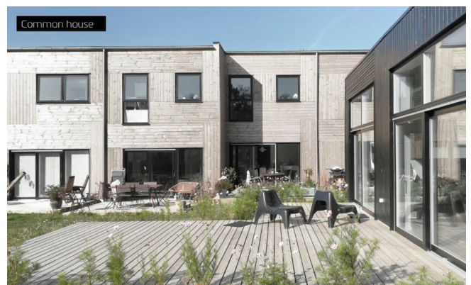
Common house and dwellings at Stavnsholthave (Source: Urban Power)
