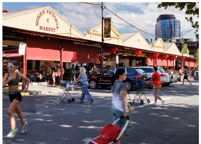
QVM Shed Restoration by NH Architecture with City of Melbourne. 2023 AIA Heritage Award Photo by Dianna Snape
