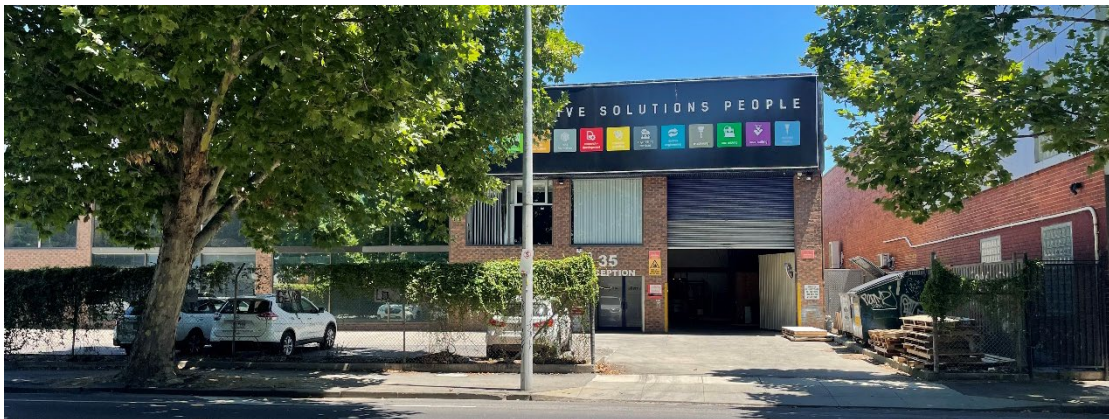
Figure 5 - View of north eastern corner of building on the subject site (where the northern link is proposed)
