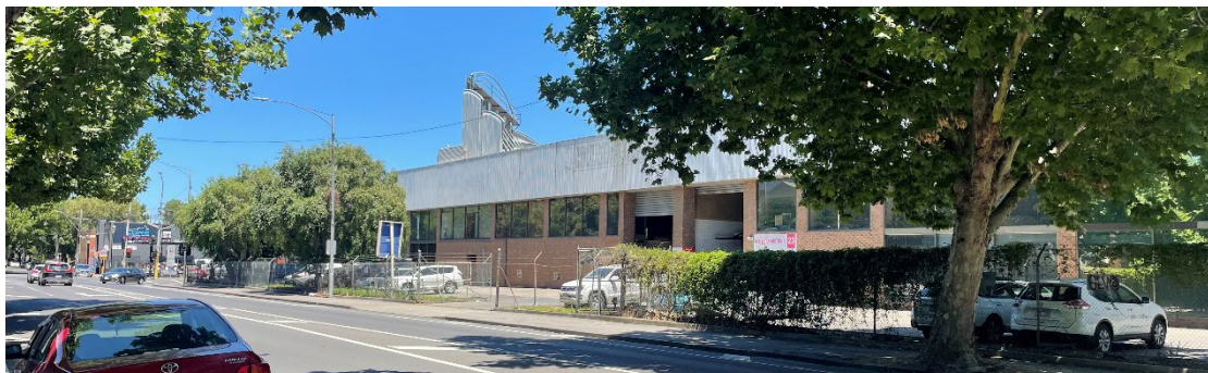
Figure 3 - Partial view of east boundary (Boundary Road) of the subject site
