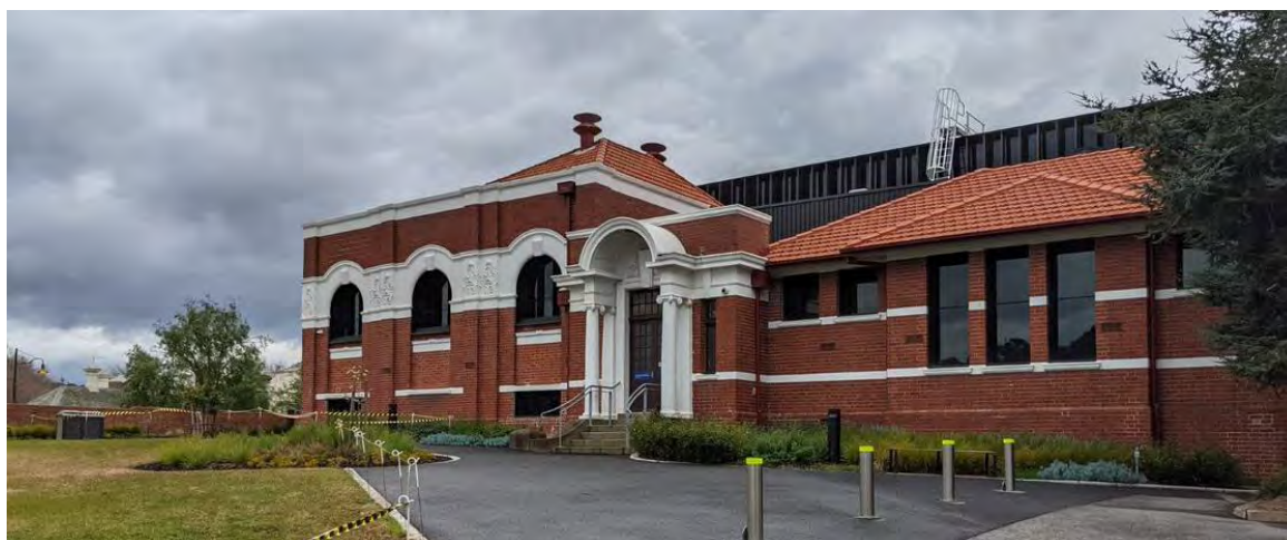
Figure 514. 1908 Veterinary College building. Note the original window frames have been replaced and a large (black) extension has been added to its rear. (Source: GML Heritage, 2022)
