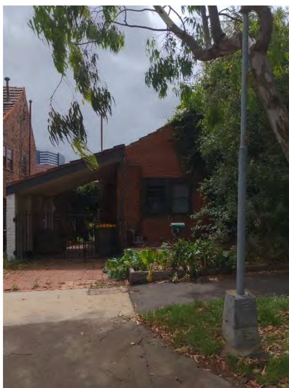
Figure 493. 7 St Georges Grove, Parkville. (Source: GML 2022)
