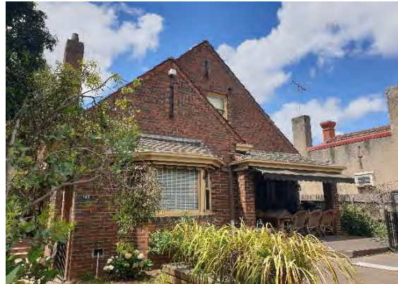
Figure 536. 130–132 Flemington Road. (Source: GML, 2022)
