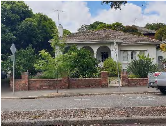
Figure 490. Front view of 30–32 Manningham Street. (Source: GML 2022)
