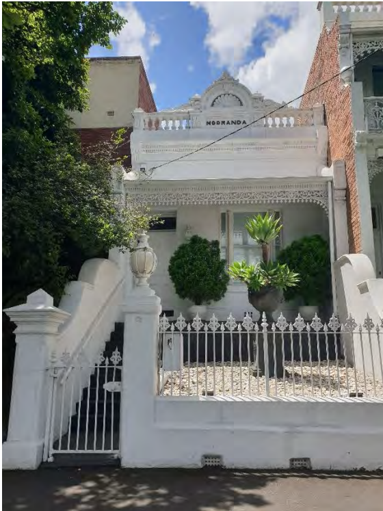
Figure 531. 78 Flemington Road. (Source: GML, 2022)
