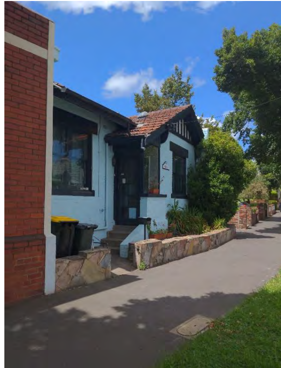
Figure 538. 100–102 Flemington Road. (Source: GML, 2022)
