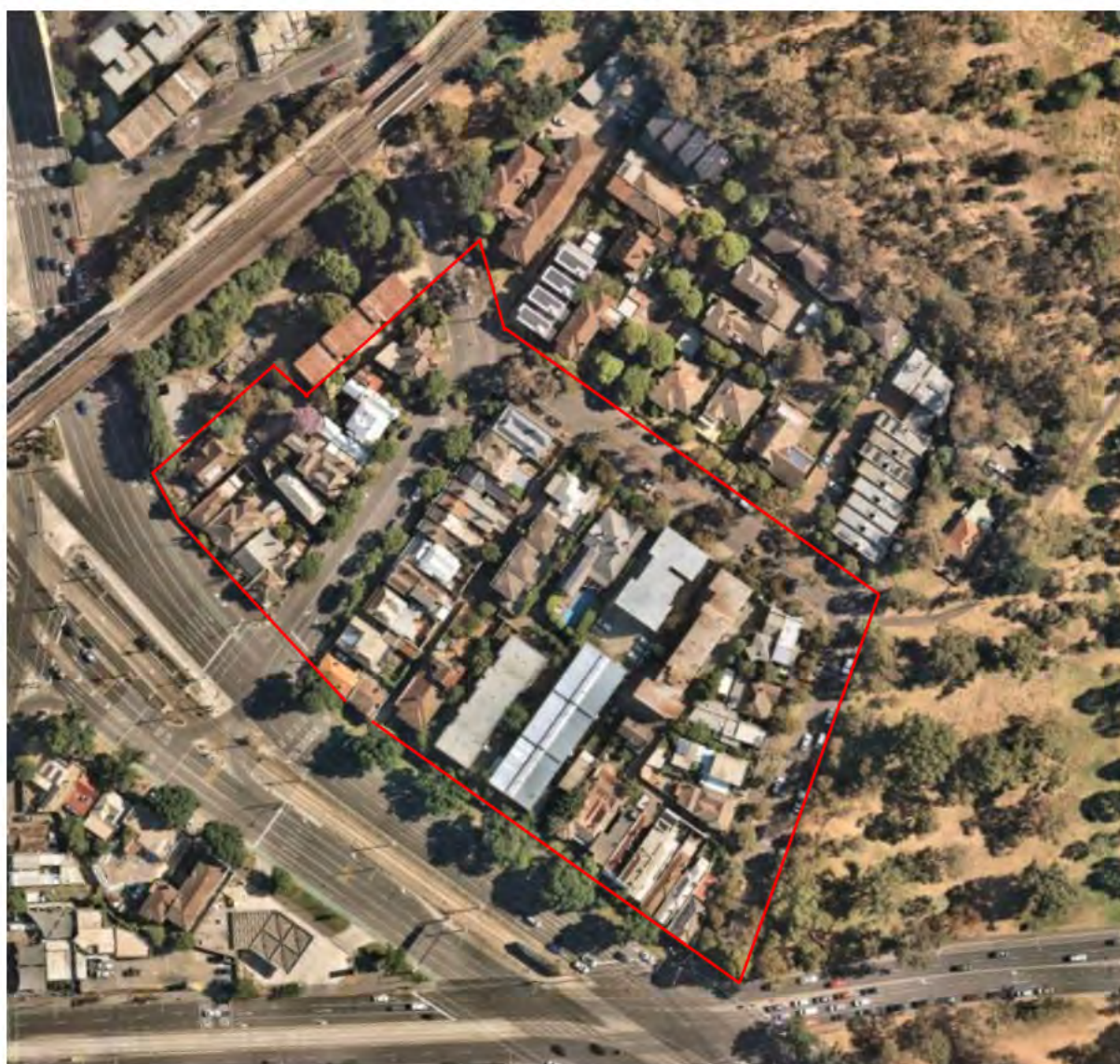
Figure 526. Aerial image of the West Parkville Precinct. (Source: Nearmap, 2023)
