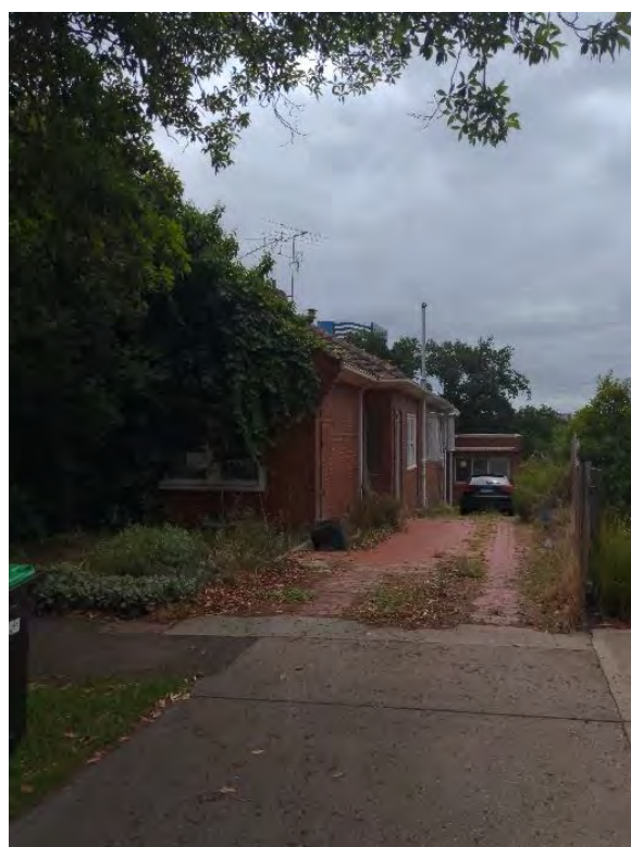
Figure 494. 9 St Georges Grove, Parkville. (Source: GML 2022)
