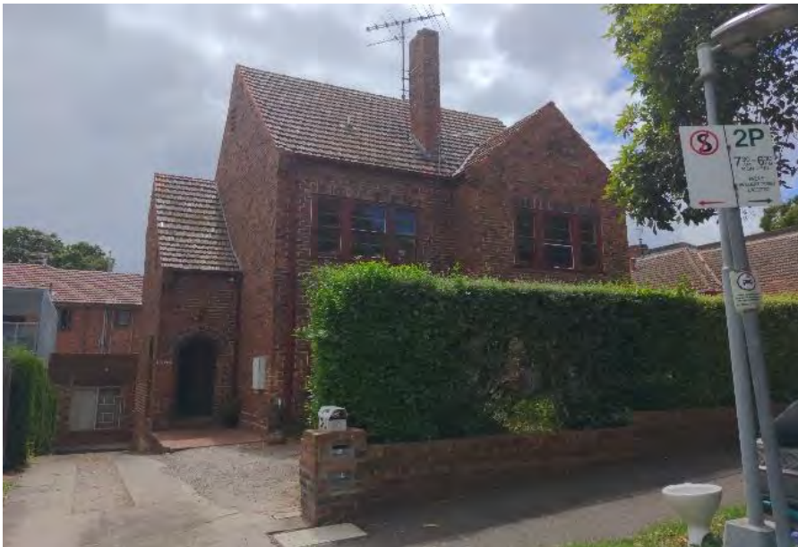
Figure 492. 1–3 St Georges Grove, Parkville. (Source: GML 2022)
