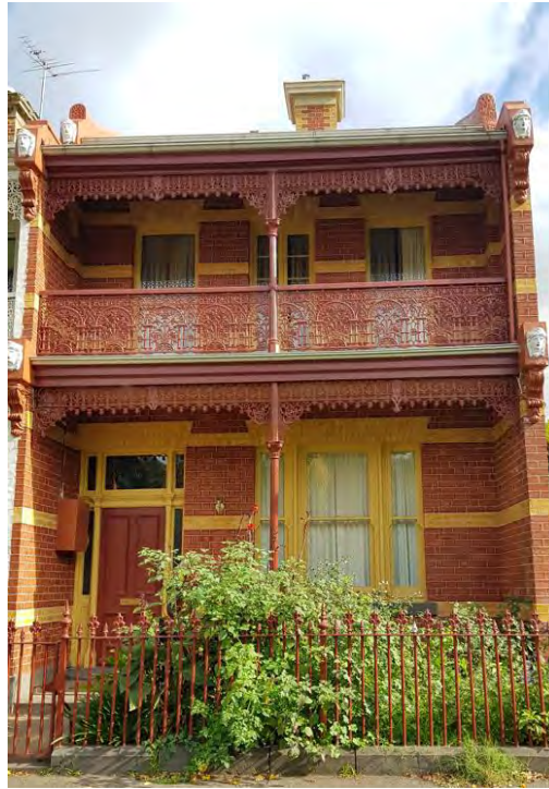
Figure 468. View of the primary eastern elevation of 549 Royal Parade. (Source: GML Heritage, 2022)
