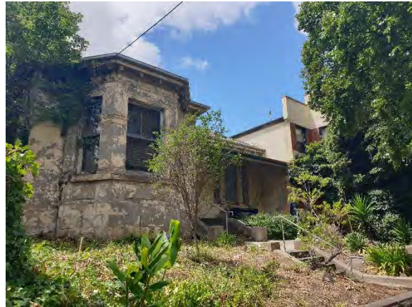
Figure 528. 80–84 Flemington Road. (Source: GML, 2022)
