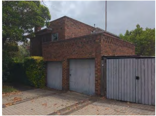
Figure 496. View of 34–40 Manningham Street, Parkville, from St Georges Grove. (Source: GML 2022)
