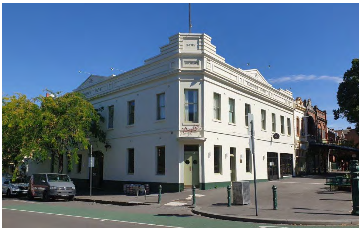
Figure 517. Naughtons Hotel, 43–49 Royal Parade, Parkville. Originally built in 1873, and extensively remodelled in 1923 by architect Robert McIntyre, the remodelled hotel incorporated two shop buildings at 47 and 49 Royal Parade. (Source: GML Heritage, 2022)
