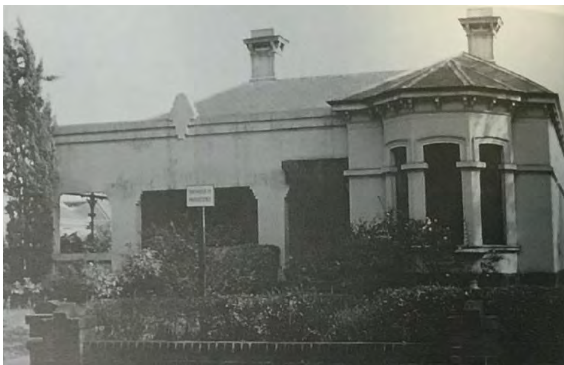
Figure 3.76. The Victorian-era residence 'Homeville' at 343 Royal Parade, adapted for use by CSIRO. (Source: The Lennox Legacy )
