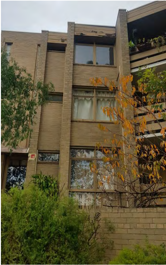
Figure 94. Detail of the primary elevation and stepped bays. (Source: GML Heritage, 2022)
