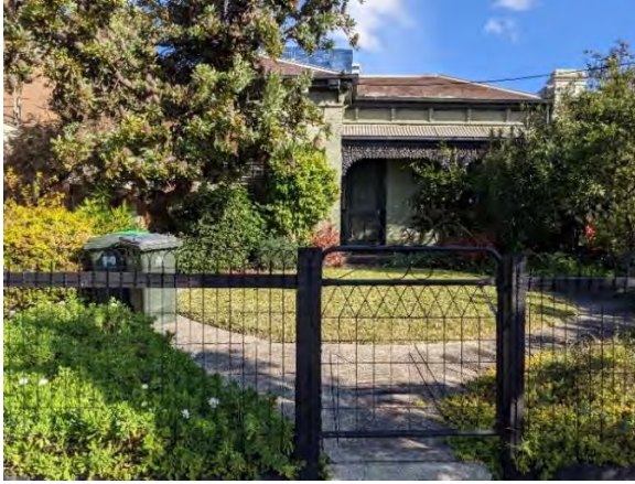
Figure 82. 121 Manningham Street, Parkville. (Source: GML, 2022)
