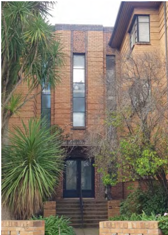
Figure 26. The western elevation of the connecting bay. (Source: GML Heritage, 2022)
