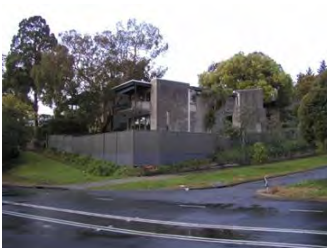
Figure 106. 76 Molesworth Street, Kew. (Source: City of Boroondara)
