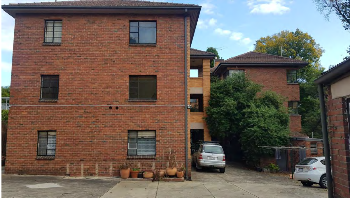
Figure 34. The eastern elevation of the building. (Source: GML Heritage, 2022)
