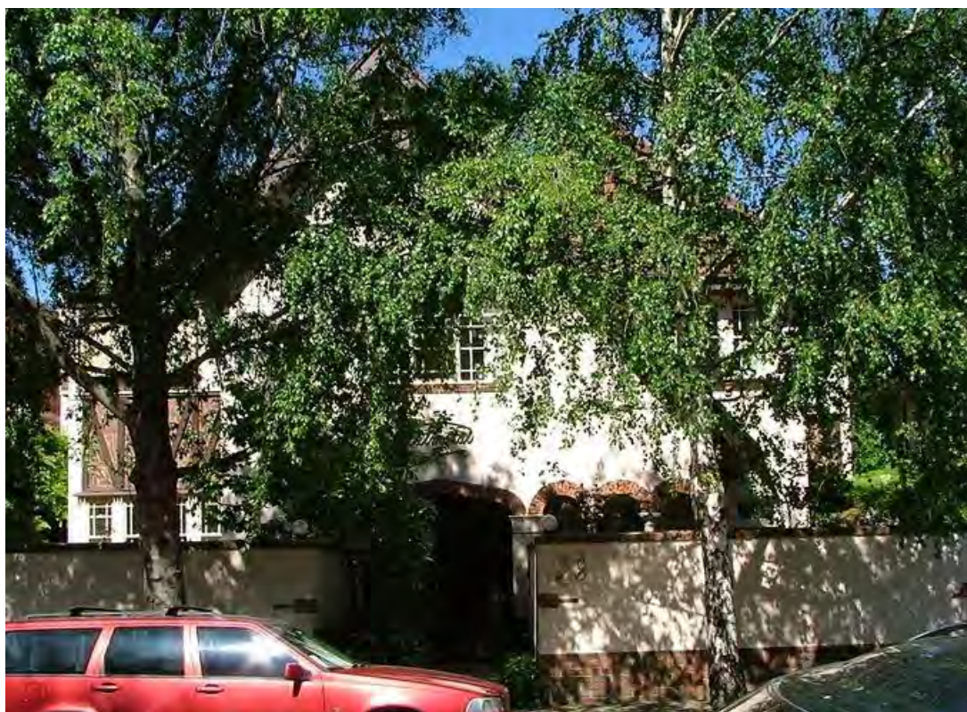
Figure 55. Balmoral at 28 Marne Street, South Yarra. (Source: City of Melbourne, via Hermes Orion)
