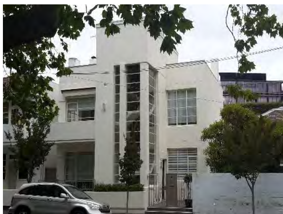
Figure 73. Yarrum Flats, 67–69 Bromby Street, South Yarra. (Source: GML, 2021–22)
