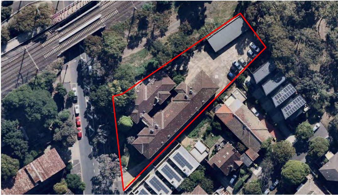
Figure 24. Aerial view of the building in April 2022, showing the irregular shape of the site, and Manningham Street to the left of the image. The approximate boundary of the property is indicated in red. (Source: Nearmap, with GML overlay)
