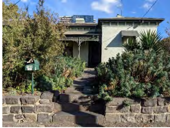
Figure 83. 123 Manningham Street, Parkville. (Source: GML, 2022)
