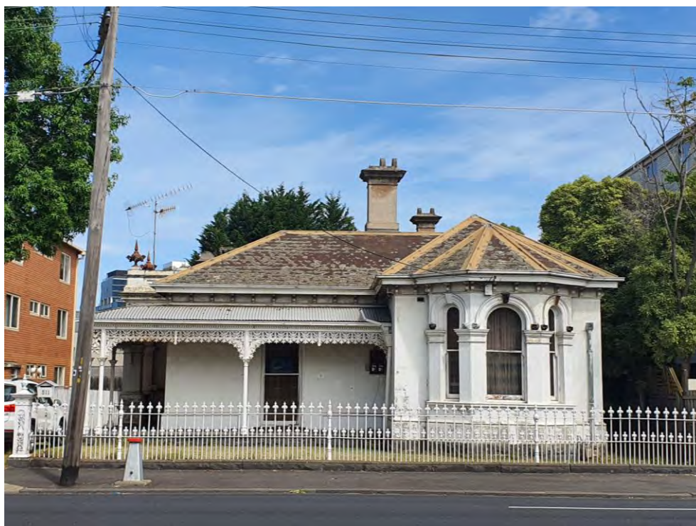
Figure 88. 507–511 Punt Road, South Yarra. (Source: GML, 2021–22)
