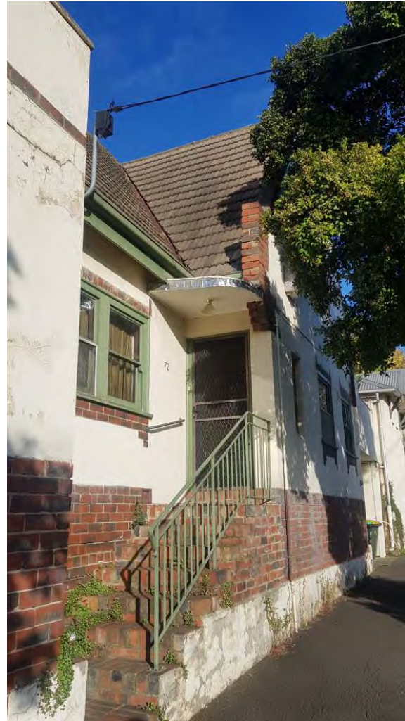
Figure 49.. View showing the primary entrance to the dwelling. (Source: GML Heritage, 2022)
