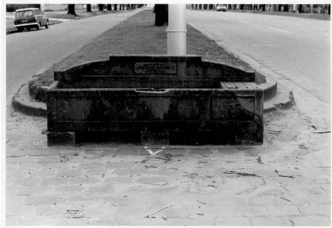
Figure 3.37. Early concrete horse trough c1890ss-1900s, possibly Royal Parade, photographed by John T Collins, [nd], c1960s. (Source: John T Collins Collection, State Library Victoria, Accession No. H98.250/1551)
