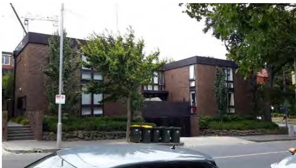
Figure 102. 'Kurneh', 2–10 Anderson Street, South Yarra. (Source: GML, 2021–22)
