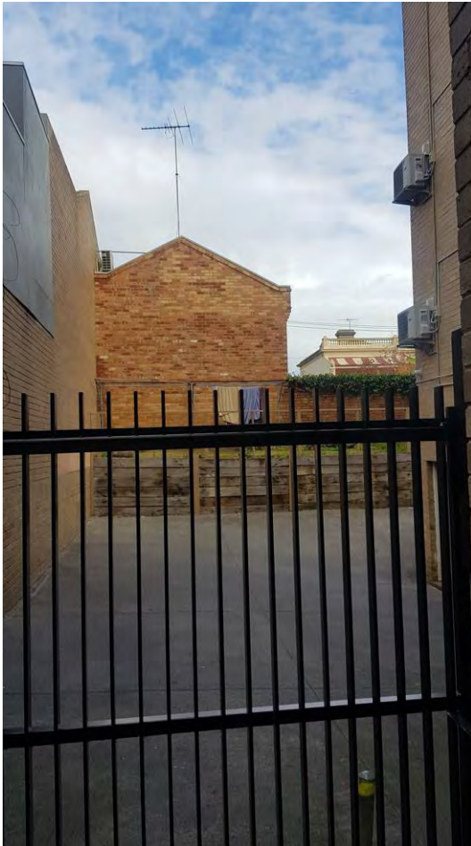
Figure 100. View towards the rear carpark area. (Source: GML Heritage, 2022)
