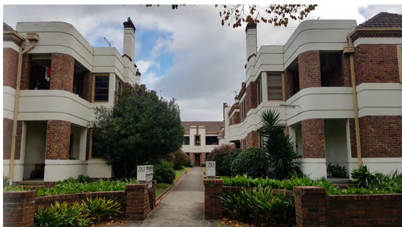
Figure 37. Park Court, 283–291 Royal Parade, Parkville. (Source: GML Heritage, 2022)
