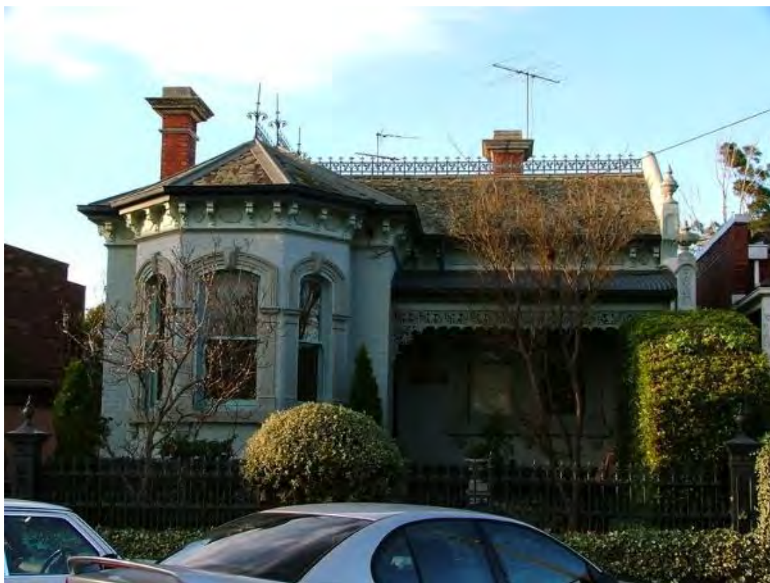
Figure 90. Daylesford, 98 Molesworth Street, North Melbourne. (Source: City of Melbourne)
