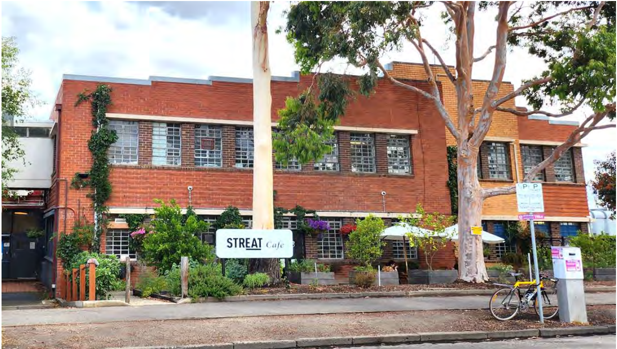
Figure 123. View of the former junior girls' and toddlers' building. (Source: GML, February 2023)
