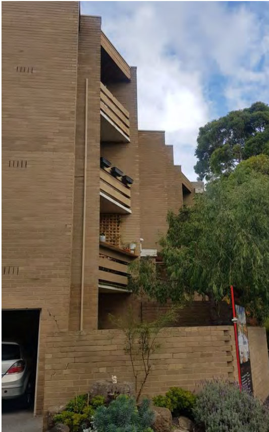
Figure 98. View across the primary elevation, showing the faceted, sculptural facade. (Source: GML Heritage, 2022)
