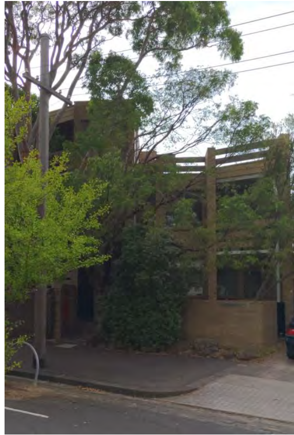
Figure 95. View towards the southern wing and the rooftop 'Sky Garden'. (Source: GML Heritage, 2022)
