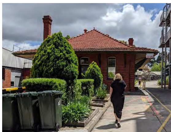
Figure 147. Jennerian Building south elevation. (Source: GML, December 2022)
