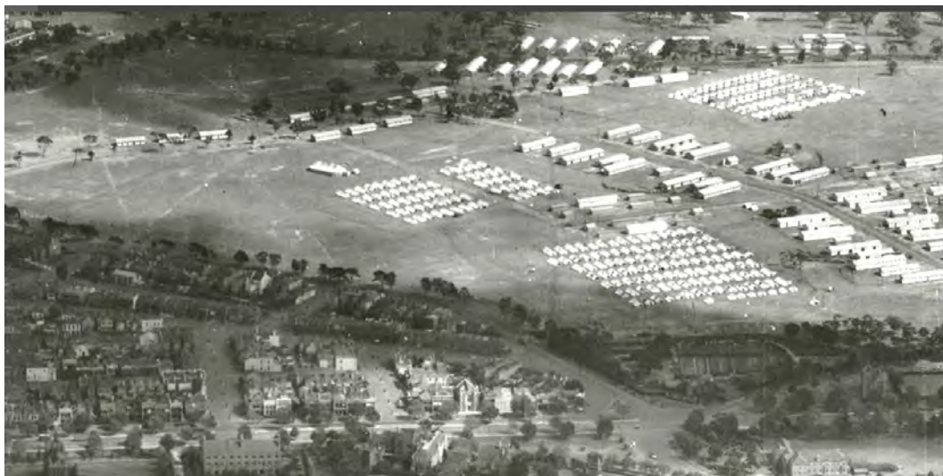
Figure 3.53. Aerial view looking west over Royal Park in 1942, showing the military camp during the Second World War. (Source: University of Melbourne Archives – Copyright restrictions may apply)
