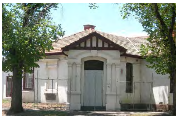
Figure 132. An early building from the Carlton Refuge. (Source: Heritage Victoria, via Hermes Orion)
