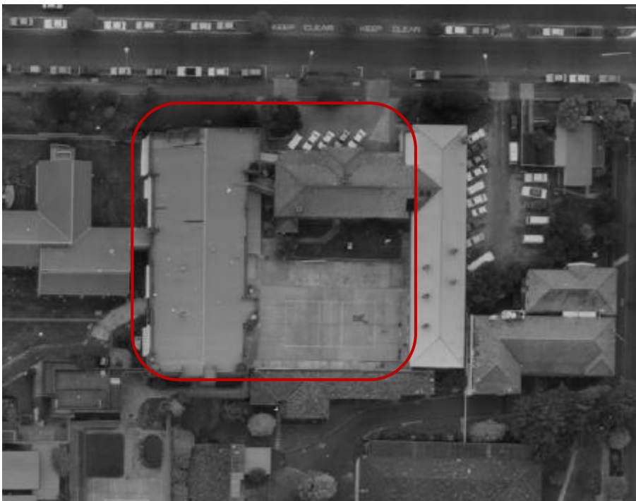
Figure 117. View showing a detail of a 1986 aerial with the 1925 nurses' quarters (right building in the area outlined in red) and 1940 junior girls' and toddlers' building (left building in the area outlined in red). (Source: LANDATA, with GML overlay)
