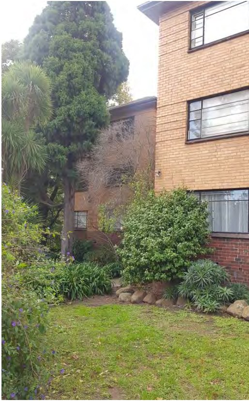
Figure 28. View across the western elevation, showing the front garden. (Source: GML Heritage, 2022)
