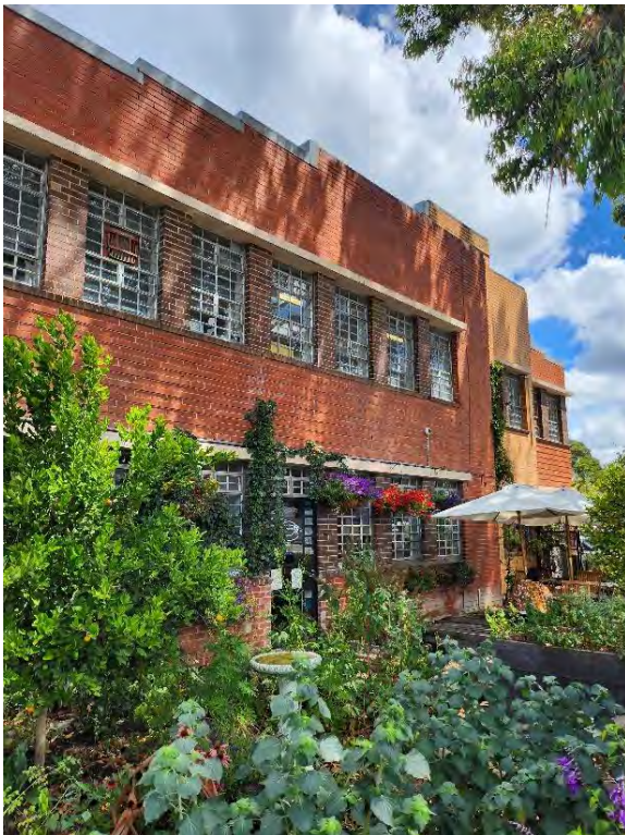
Figure 124. View of the primary elevation with a new central opening on the ground level. (Source: GML, February 2023)
