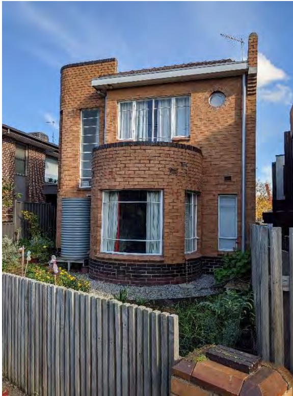
Figure 68. Front (east) elevation of the subject site. (Source: GML, 2022)
