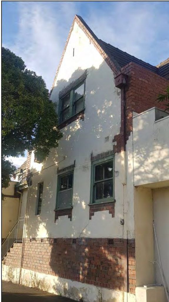
Figure 48. View showing the southwestern gable bay along the primary western elevation. (Source: GML Heritage, 2022)
