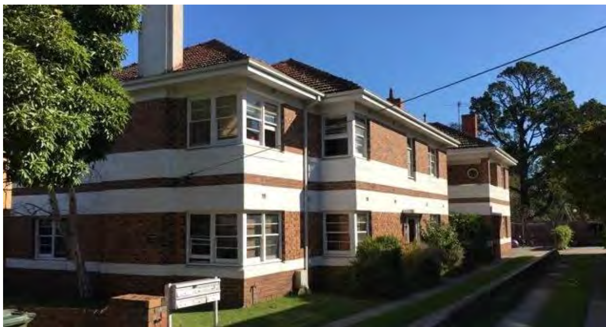
Figure 38. The flats at 43 and 45 Westbury Street, St Kilda East. (Source: City of Port Phillip, via Hermes Orion, 199766)
