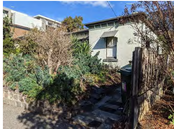
Figure 85. View of 123 Manningham Street, Parkville. (Source: GML, 2022)
