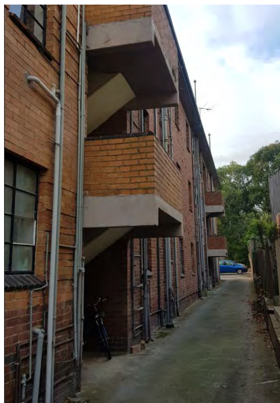
Figure 36. The southern elevation and driveway. (Source: GML Heritage, 2022)
