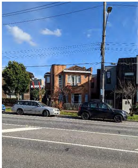
Figure 71. View of subject site from Manningham Street. (Source: GML, 2022)
