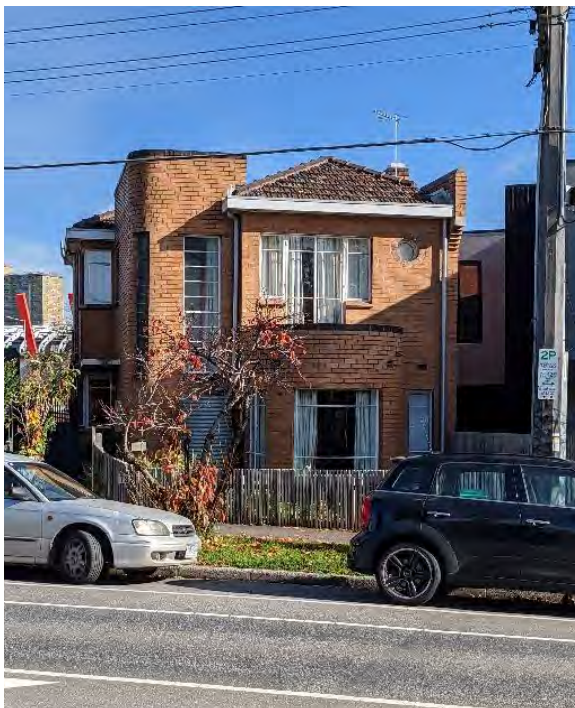
Figure 70. View of subject site from Manningham Street. (Source: GML, 2022)
