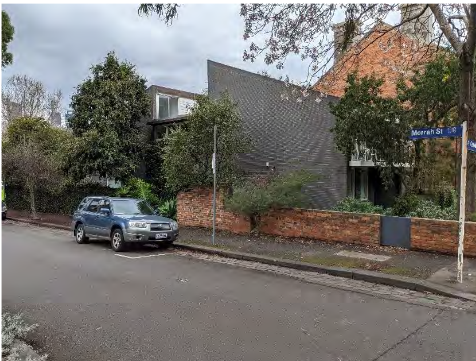
Figure 13. View of the Saunders House from Morrah Street. The rear elevation of the house is similar to the Gatehouse Street façade. The house has timber-framed windows throughout, and the balconies feature white-painted metal balustrades. (Source: GML, September 2022)
