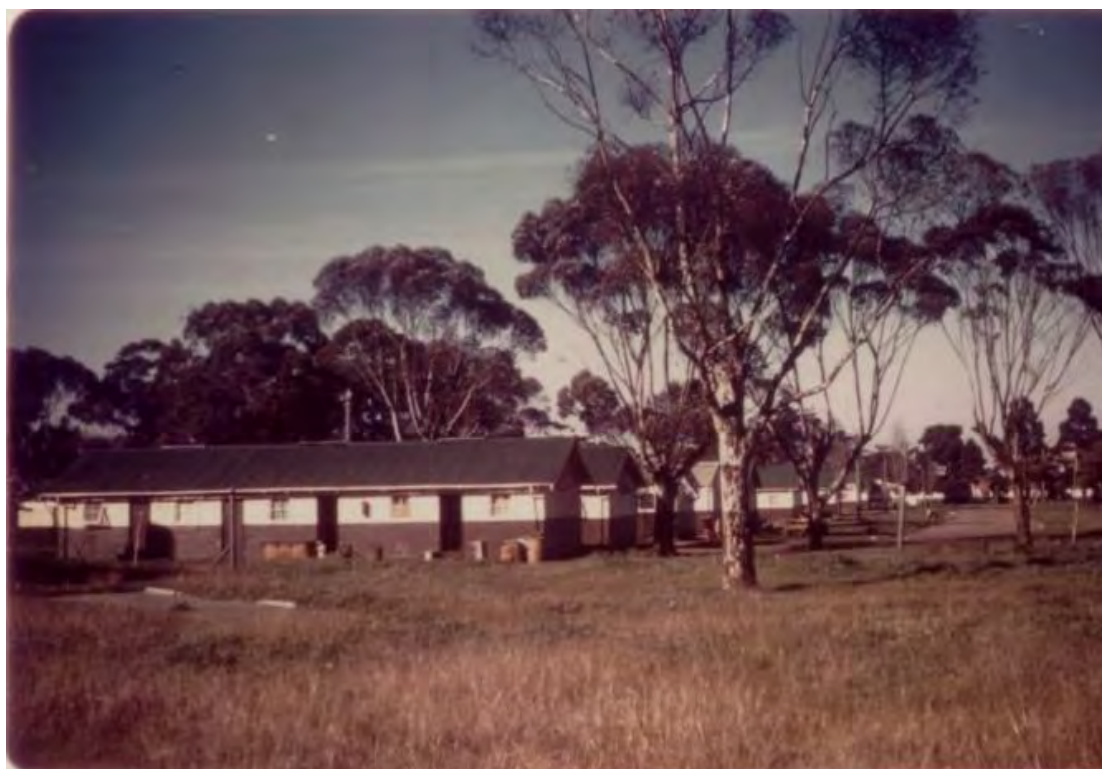
Figure 3.75. Former army barracks at Royal Park were used for emergency public housing at Camp Pell, c1950s. (Source: Melbourne Library Service)
