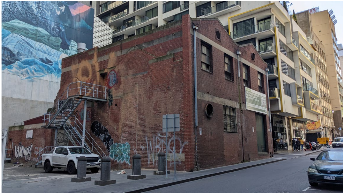
Figure 4: 620-632 Little Bourke Street, Melbourne (view from west on Little Bourke Street)
