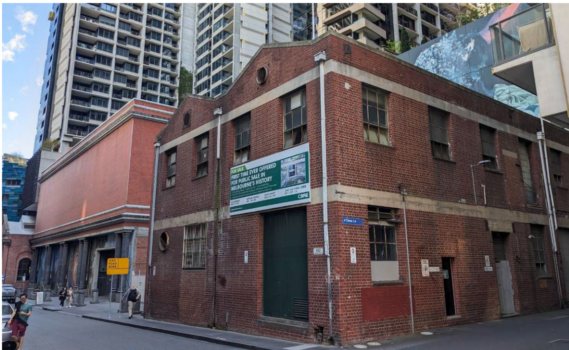
Figure 3: 620-632 Little Bourke Street, Melbourne (view from east on Little Bourke Street)
