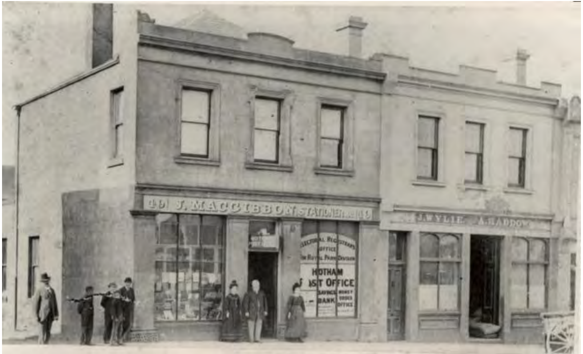
Figure 45 First Hotham Post Office, 518-520 Queensberry Street, 1860s Source: 18895, City of Melbourne Libraries
