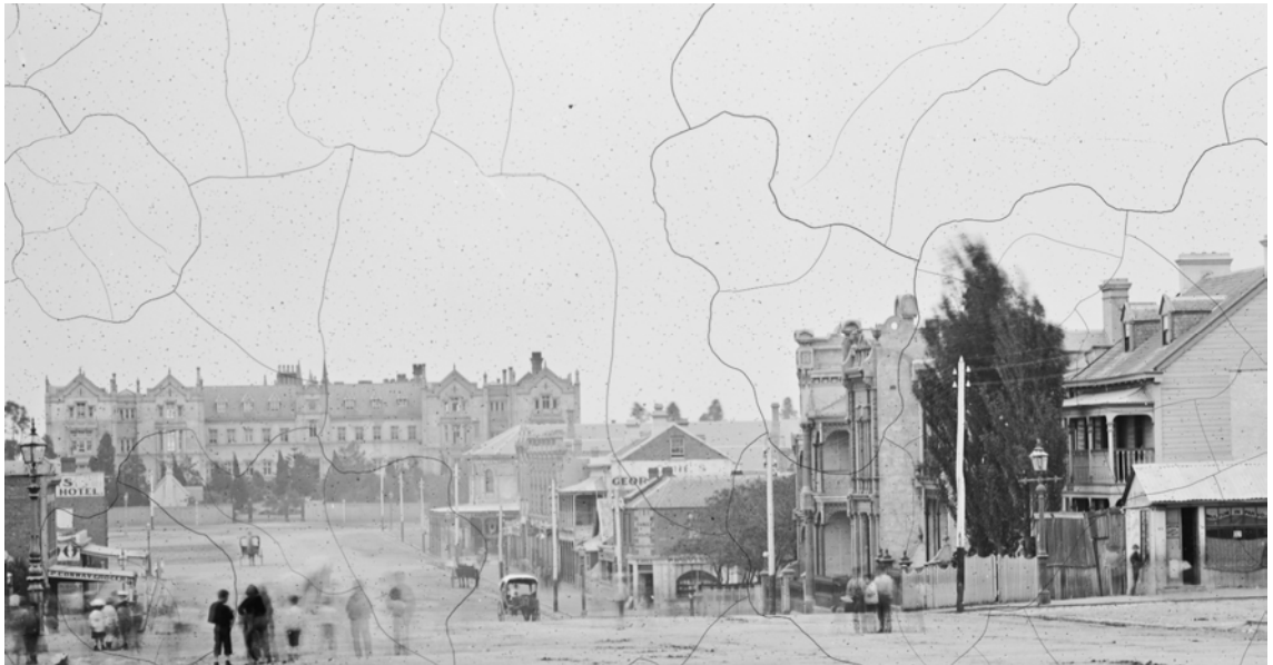
Figure 42 View west down Victoria Street from Chetwynd Street towards the Benevolent Asylum, c. 1875 Source: FL1249178, American & Australasian Photographic Company, State Library of New South Wales
