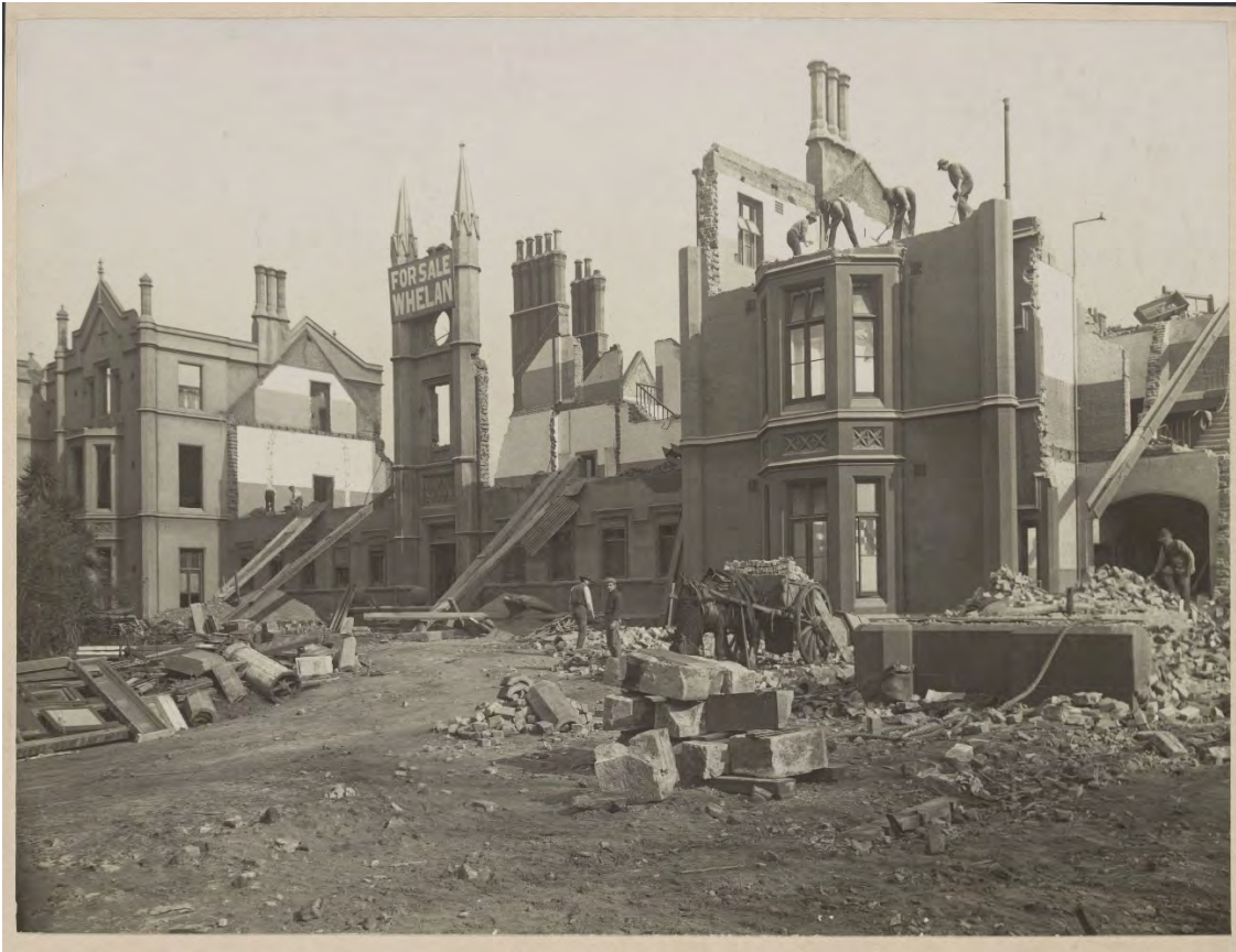
Figure 50 Whelan the Wrecker demolishing the Benevolent Asylum buildings, 1911 Source: Sydney Arnold & Co, H35792, State Library of Victoria
