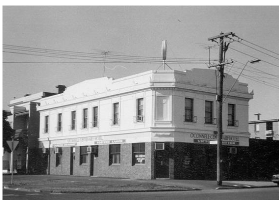
Figure 18 O'Connell's Hotel, 407 Coventry Street, South Melbourne, c. 1926
