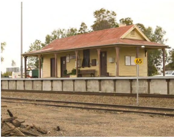
Figure 14 Dingee railway Station
