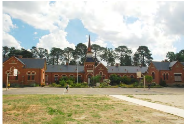
Figure 20 Beechworth Primary School No. 1560 (VHR H1718)
