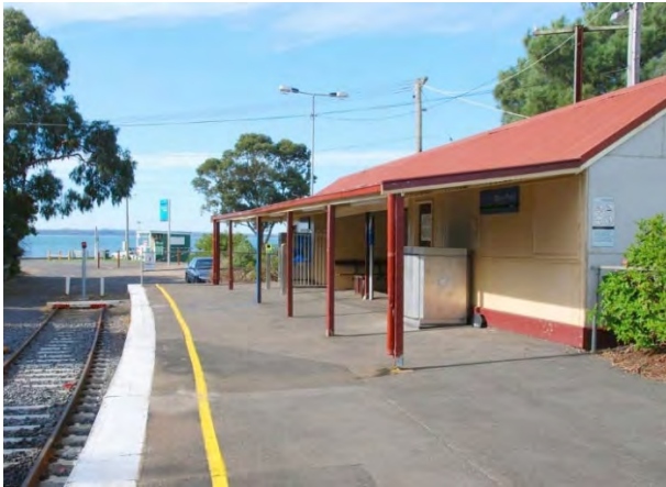
Figure 12 Crib Point Railway Station
