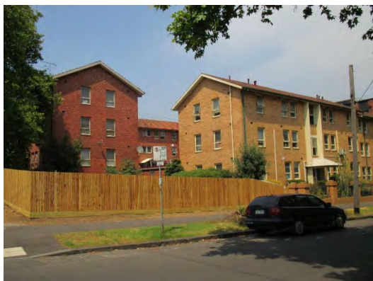
Figure 22 Arden Street Housing Commission Estate, North Melbourne, HCV completed c. 1955
