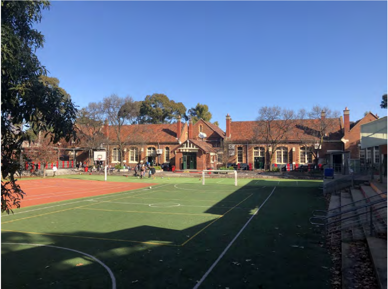
Figure 11 Rear (north) elevation of school
