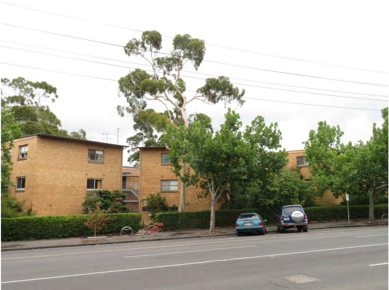
Figure 10 View of Hotham Gardens – Stage 1 from Arden Street, with angled blocks and central stairwell visible
