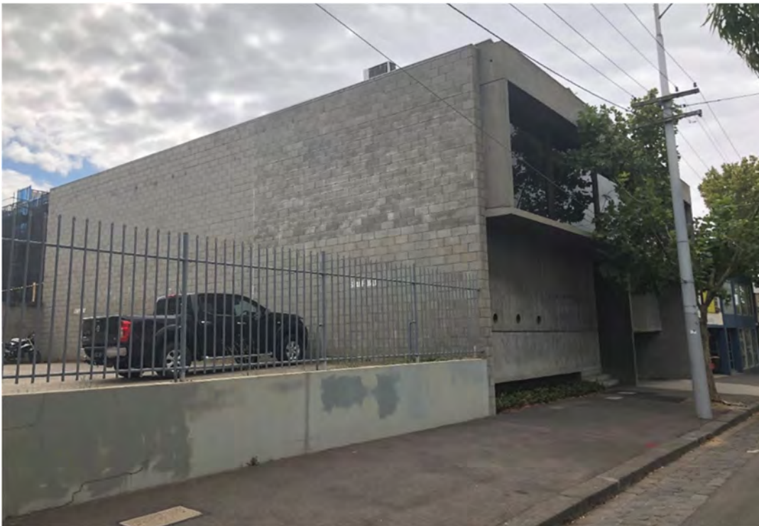
Figure 3 Former Wes Lofts office viewed from the south-east
