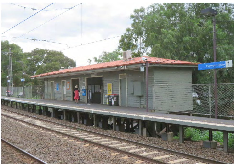
Figure 7 Flemington Bridge Station, south (up side) building
