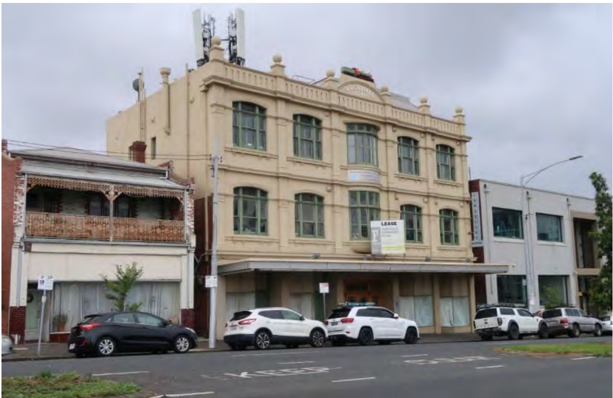
Figure 12 Loco Hall, Victoria Street
