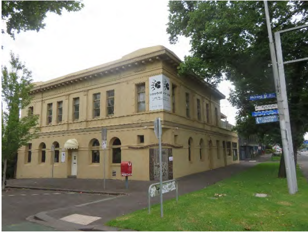
Figure 14 Former Melrose Hotel, 191-195 Melrose Street, c.1924
