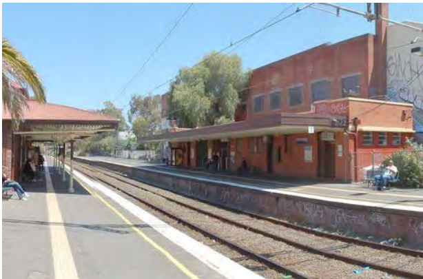
Figure 10 Prahlan Railway Station
