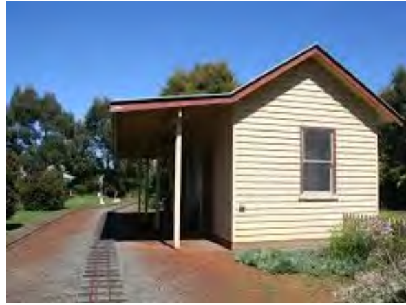
Figure 13 Cobden Railway station, preserved as part of miniature railway
