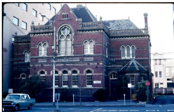
Figure 16 Former State School no. 2365, Queensberry Street, Carlton (VHR H0970)
