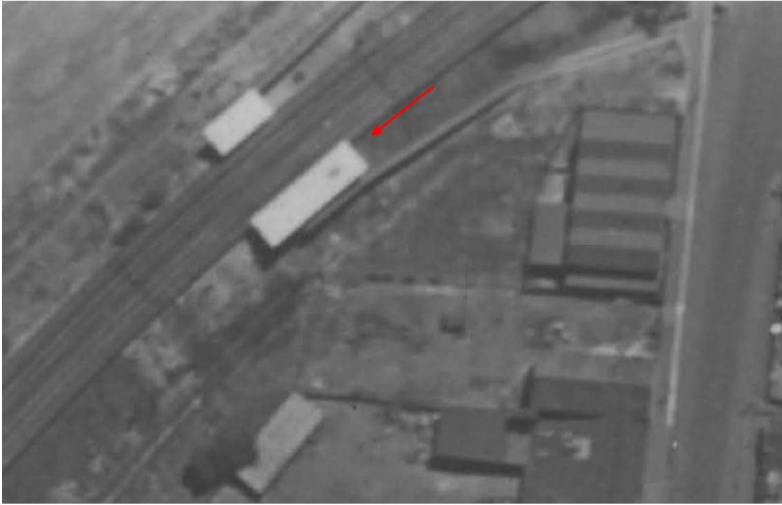
Figure 5 Aerial photograph of 1945 showing completed Flemington Bridge Railway Station complex. 'Up' side station building indicated
