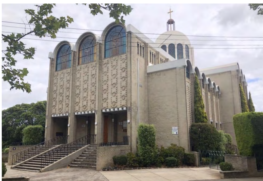
Figure 5 North and east elevations of the cathedral with the expressive vaults of the nave extending over the entrance porch and smaller vaulted transepts.
