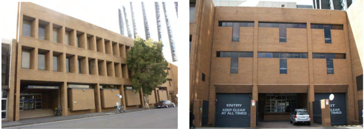
Figure 6 Former Ramsay Surgical Precinct, 182-210 Berkeley Street, Carlton, 1965-74 (HO1120). Northern end (left), Southern end (right)
