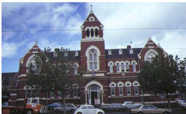
Figure 15 Former State School No. 307, Queensberry Street, North Melbourne, 1985 (H1633)
