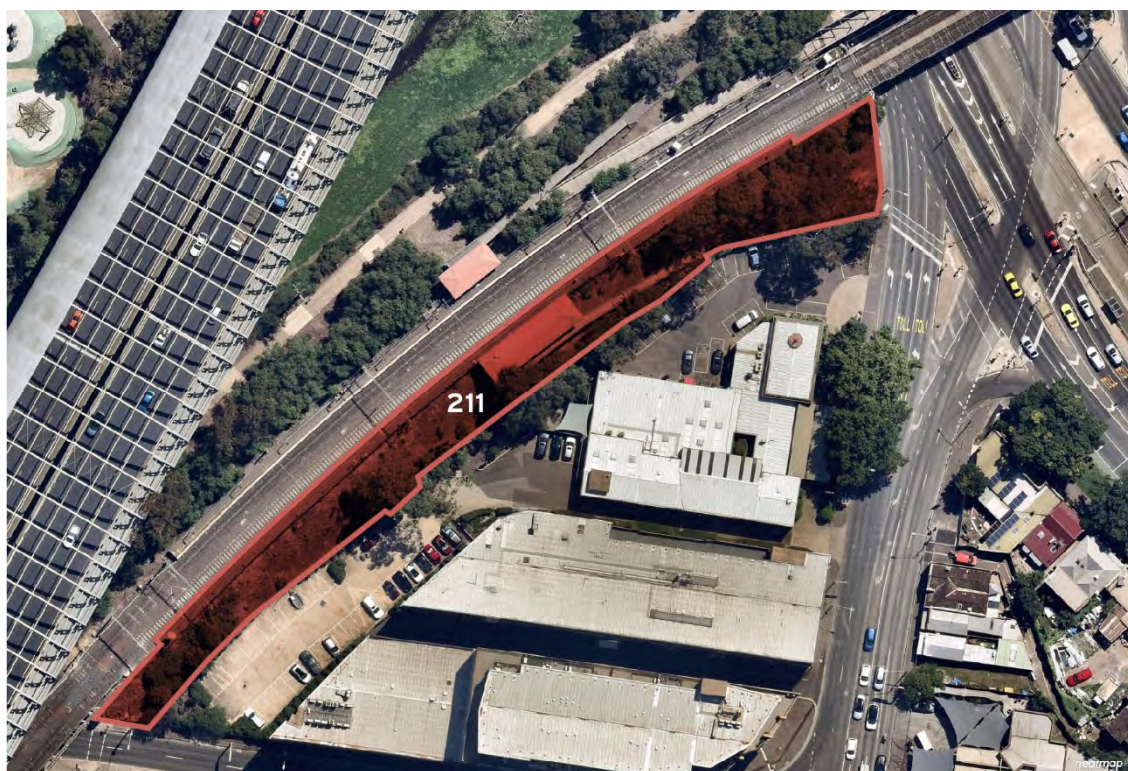
Figure 16 Aerial photograph of Flemington Bridge Railway Station, with the proposed extent of overlay indicated
