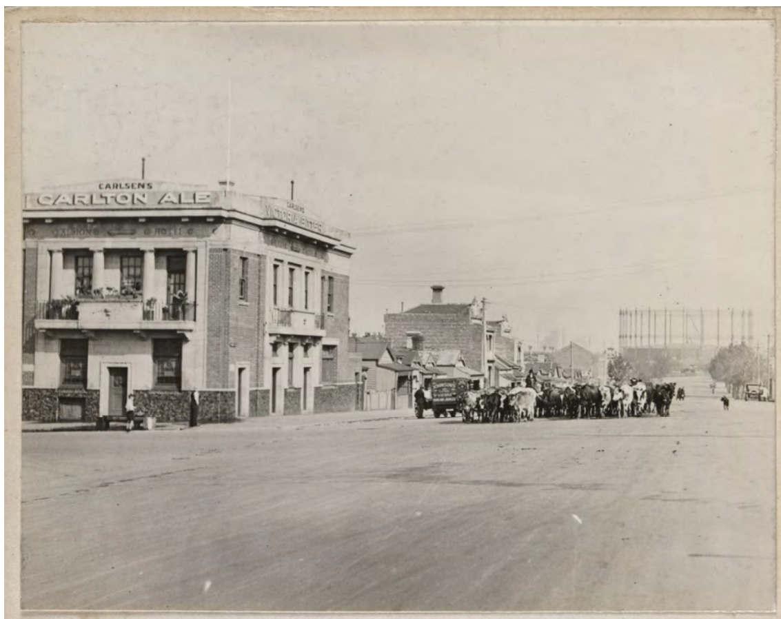
Figure 60 View west along Haines Street of the Albion Hotel, as rebuilt in 1926, in 1935 Source: H2001.291_62, State Library of Victoria
