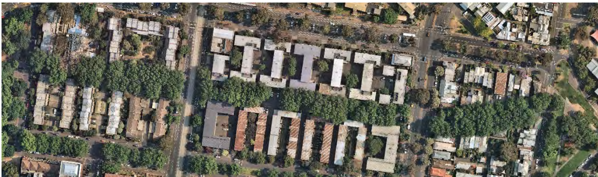
Figure 11 Recent aerial photograph showing full extent of the tree avenue
