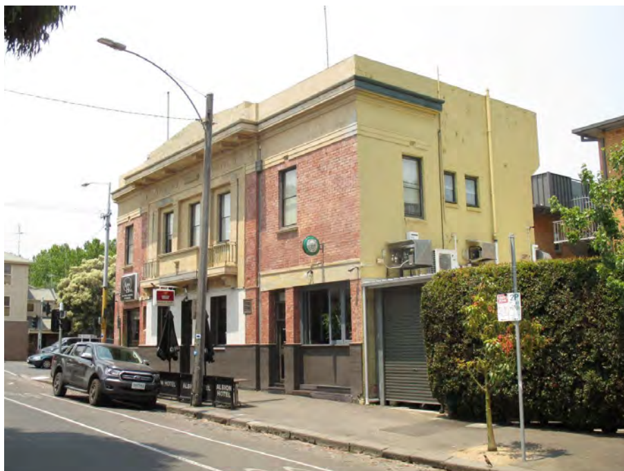
Figure 11 Albion Hotel viewed from the north-west
