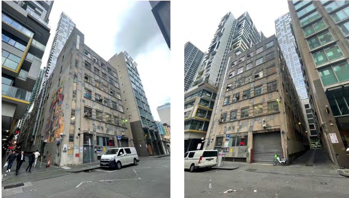
Figure 2 – View of the Site from the corner of Little Bourke Street and Rose Lane (left) and Pender Alley (right) (Source: Officer).
