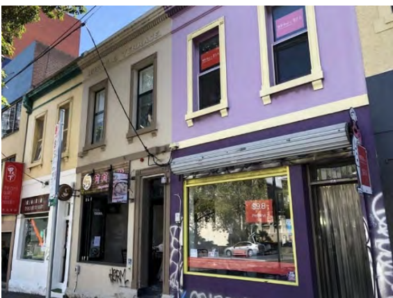
Figure 12 Russell Terrace, 68-72 Victoria Street, Carlton (HO118) Source: Lovell Chen
