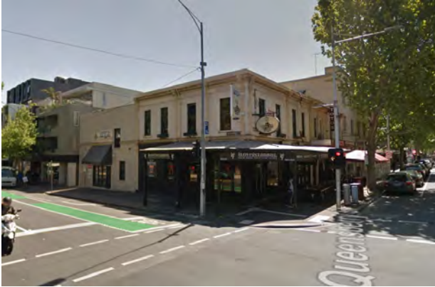
Figure 9 86-92 Queensberry Street, Carlton (HO1) Source: Google Streetview
