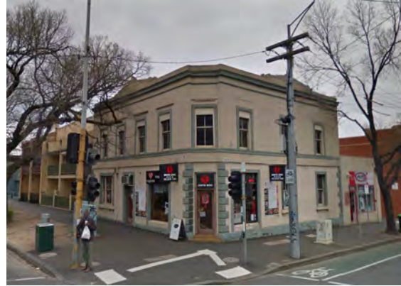
Figure 10 832 Swanston Street, Carlton (HO1) Source: Google Streetview
