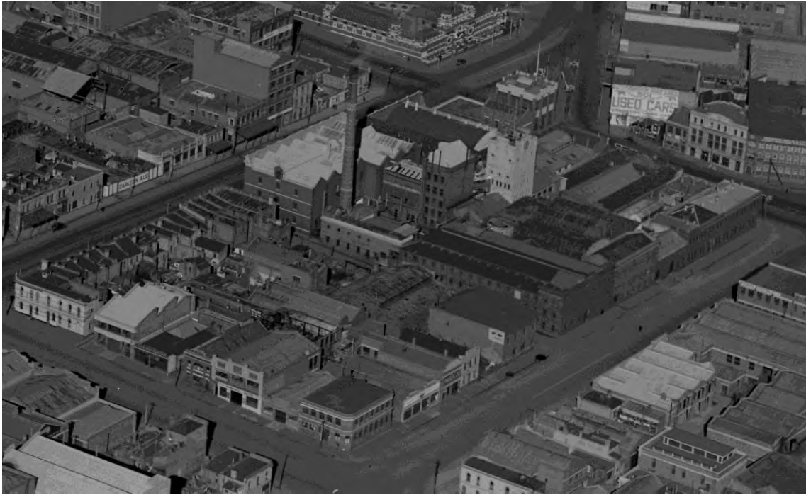
Figure 21 Oblique aerial view of the Carlton Brewery site, looking from Queensberry Street towards the Melbourne City Baths (centre top of image), 1938 Source: Airspy collection, H91.160/513, State Library of Victoria
