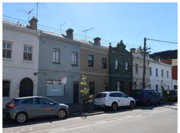
Figure 11 101-111 Cardigan Street, Carlton (HO30) Source: Lovell Chen
