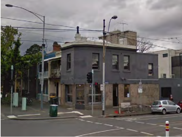
Figure 15 332 Cardigan Street, Carlton (HO1) Source: Google Streetview
