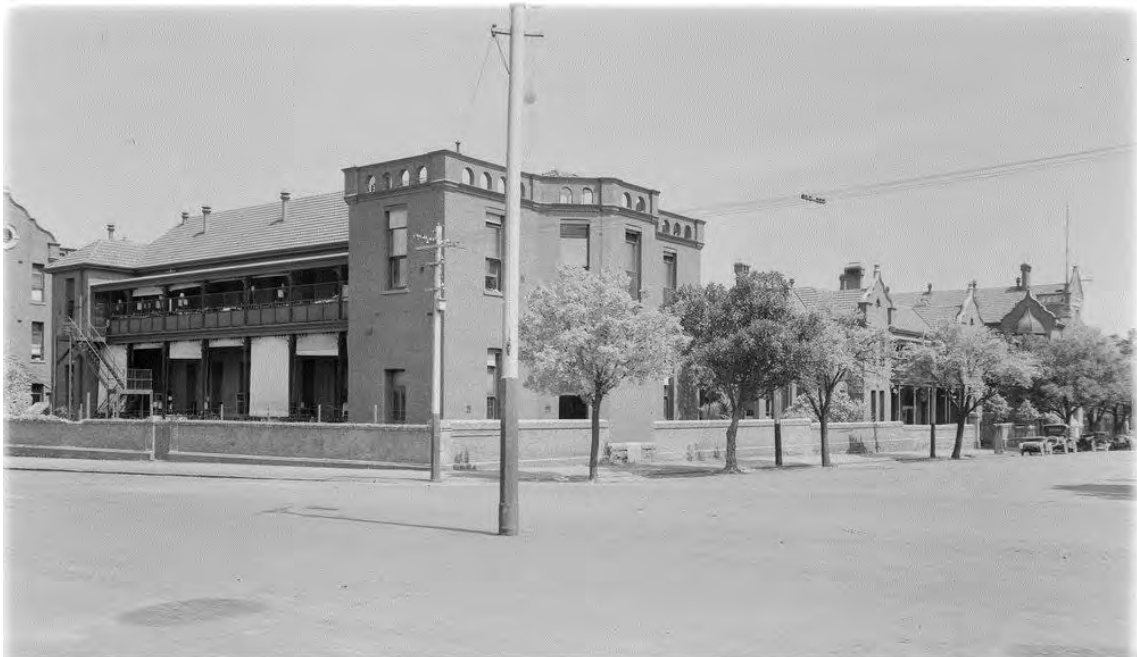
Figure 42 c.1920s-40s Rose Postcard photograph of Children's Hospital, at intersection of Rathdowne and Pelham streets; the building in the foreground was demolished in the 1990s; the Administration Building and Princess May Pavilion are at right. Source: State Library of Victoria.
