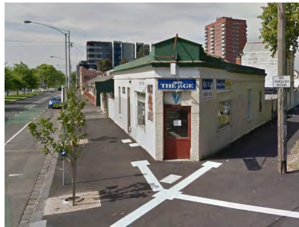
Figure 12 30 Canning Street, Carlton (HO1) Source: Google Streetview
