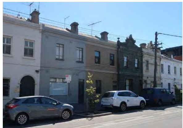
Figure 11 101-111 Cardigan Street, Carlton (H030) Source: Lovell Chen
