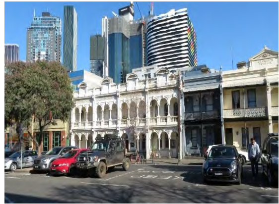
Figure 9 51-65 Cardigan Street, Carlton (HO27) Source: Lovell Chen
