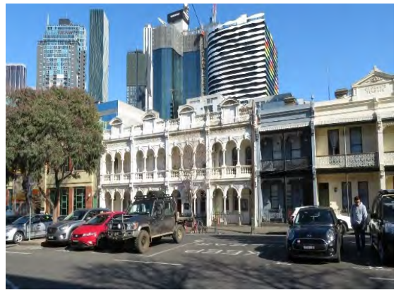
Figure 9 51-65 Cardigan Street, Carlton (HO27) Source: Lovell Chen
