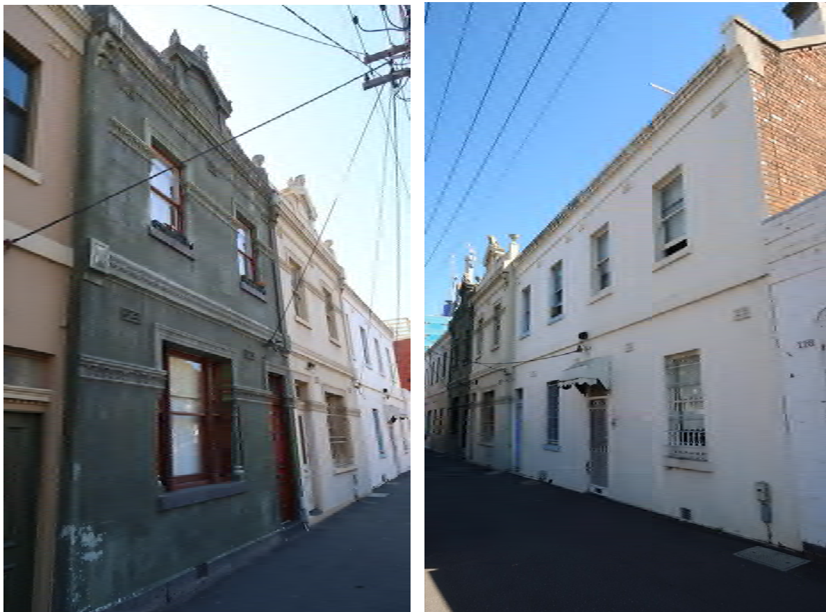
Figure 7 Remodelled facades at nos 105-107 Cardigan Street (at left); 101-111 Cardigan Street viewed from the north
