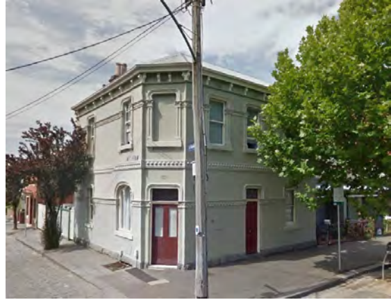
Figure 7 Former hotel at 68-70 Kay Street, Carlton (HO1) Source: Streetview
