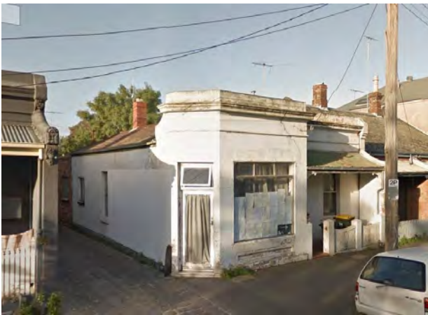
Figure 11 76 Palmerston Street, Carlton (HO1) Source: Google Streetview
