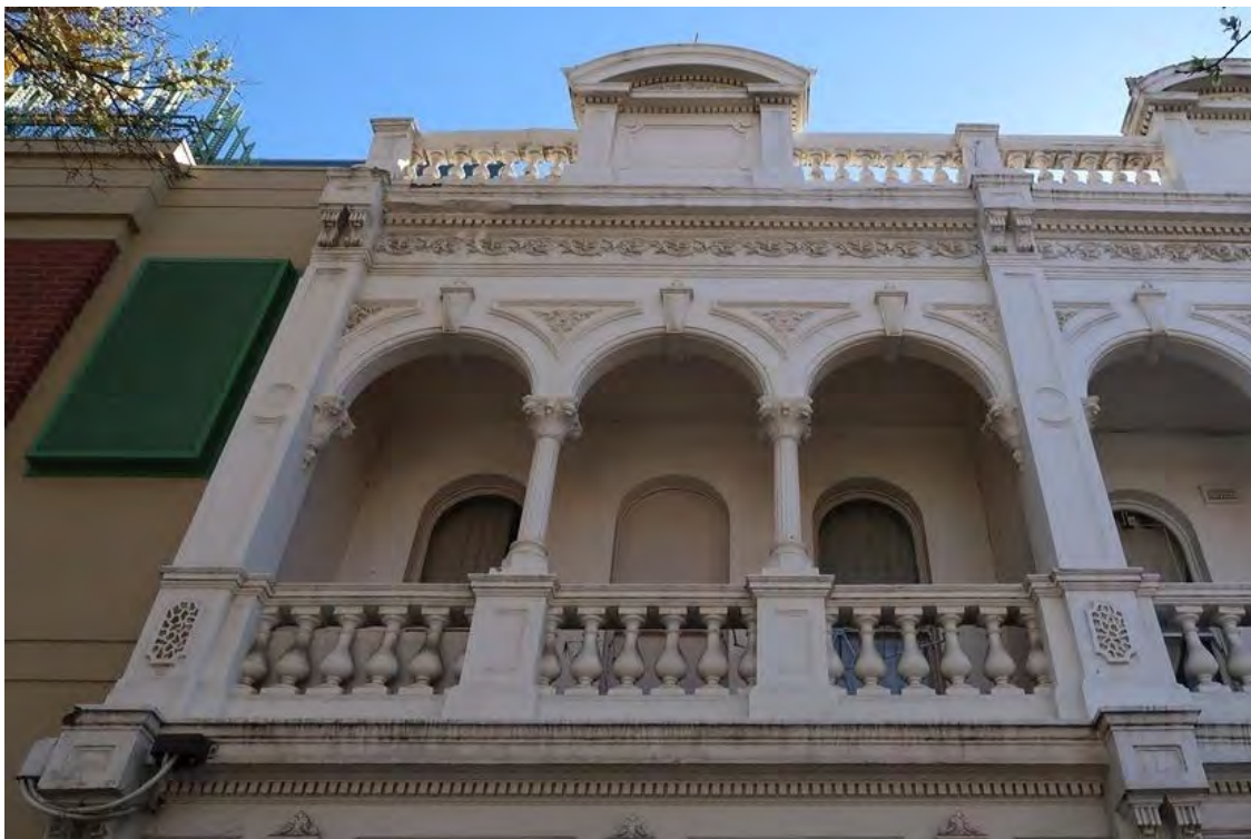
Figure 6 Upper façade, 51 Cardigan Street, Carlton
