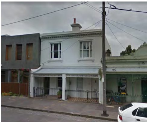
Figure 12 36 Macarthur Place North (HO1) Source: Streetview
