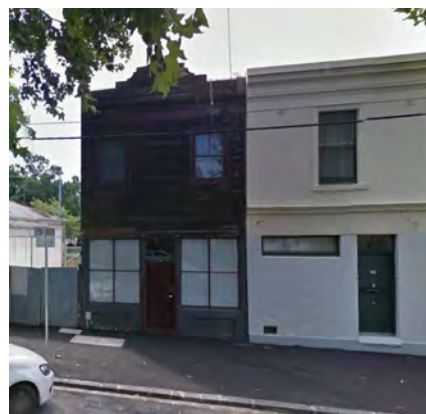
Figure 14 68 Barkly Street, Carlton (HO1) Source: Google Streetview
