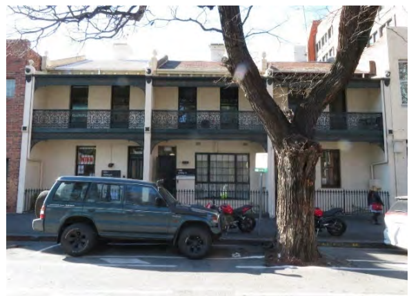
Figure 13 18-22 Cardigan Street, Carlton (HO35) Source: Lovell Chen
