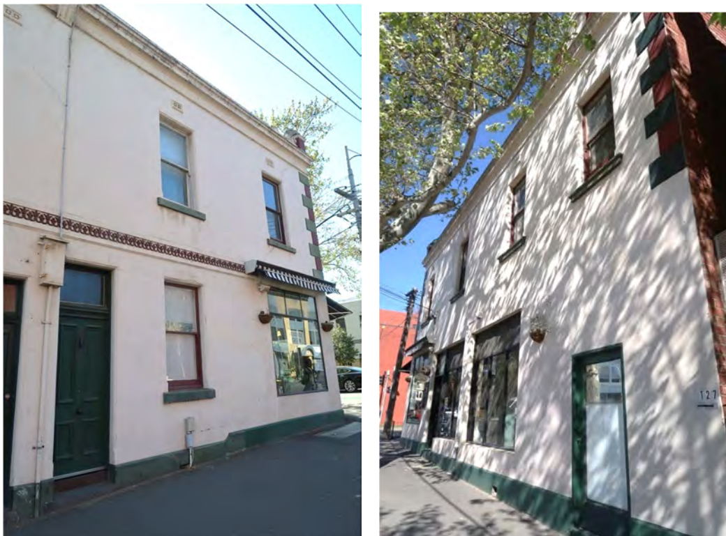
Figure 8 Nos 83-87 Cardigan Street; Cardigan Street façade (at left); Queensberry Street facade (at right) Source: Lovell Chen
