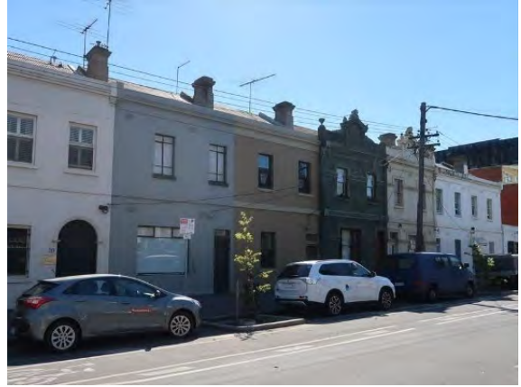
Figure 13 101-111 Cardigan Street, Carlton (HO30) Source: Lovell Chen
