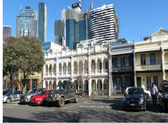
Figure 9 51-65 Cardigan Street, Carlton (HO27) Source: Lovell Chen
