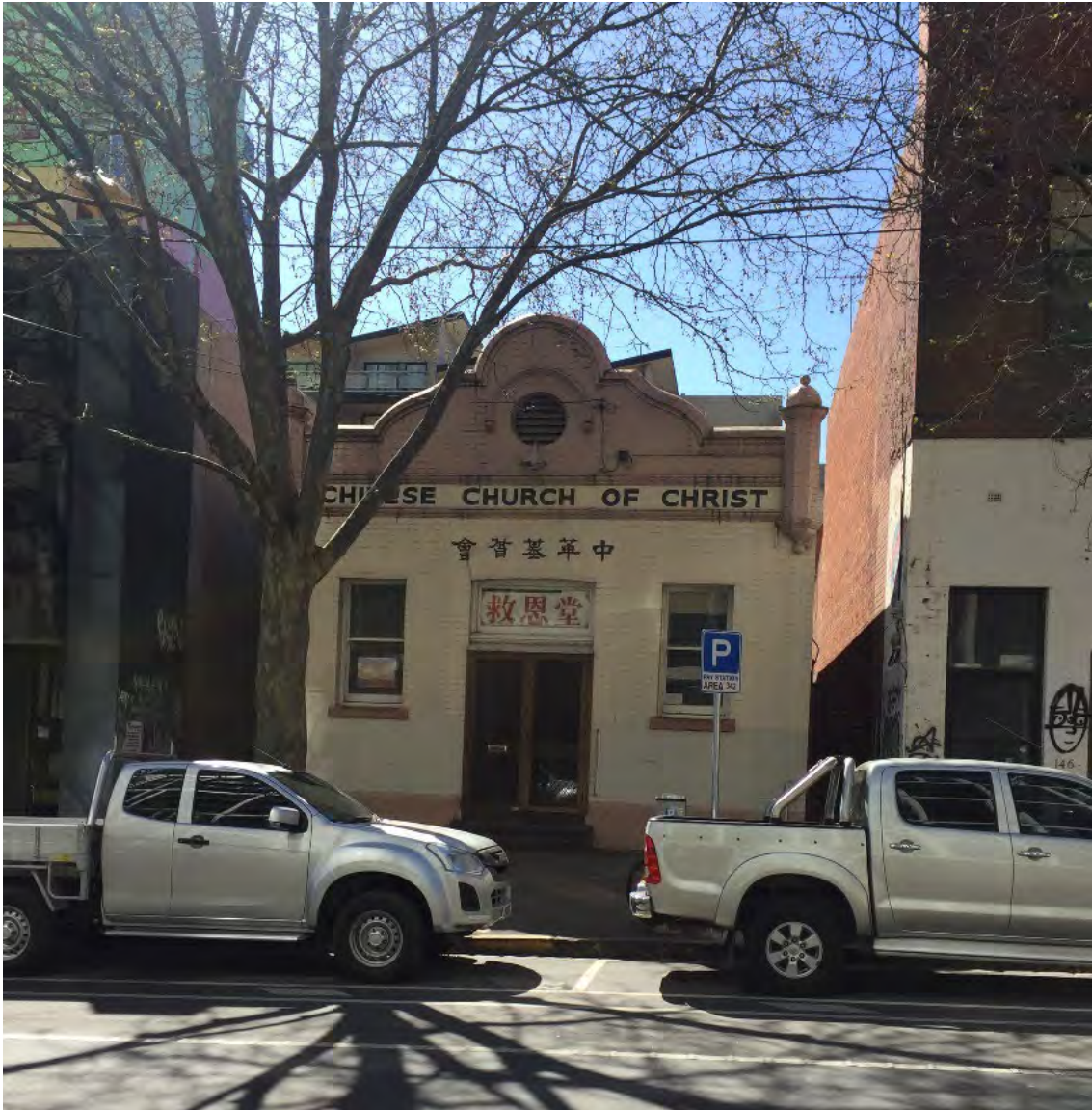
Figure 1 2018 view of the Chinese Mission Church from the south in Queensberry Street Source: Lovell Chen
