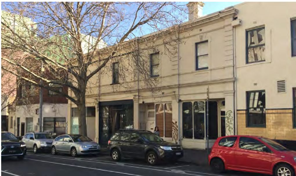
Figure 12 View of Hotel Lincoln and Environs Precinct to Queensberry Street, with hotel (part) at right and church at left Source: Lovell Chen
