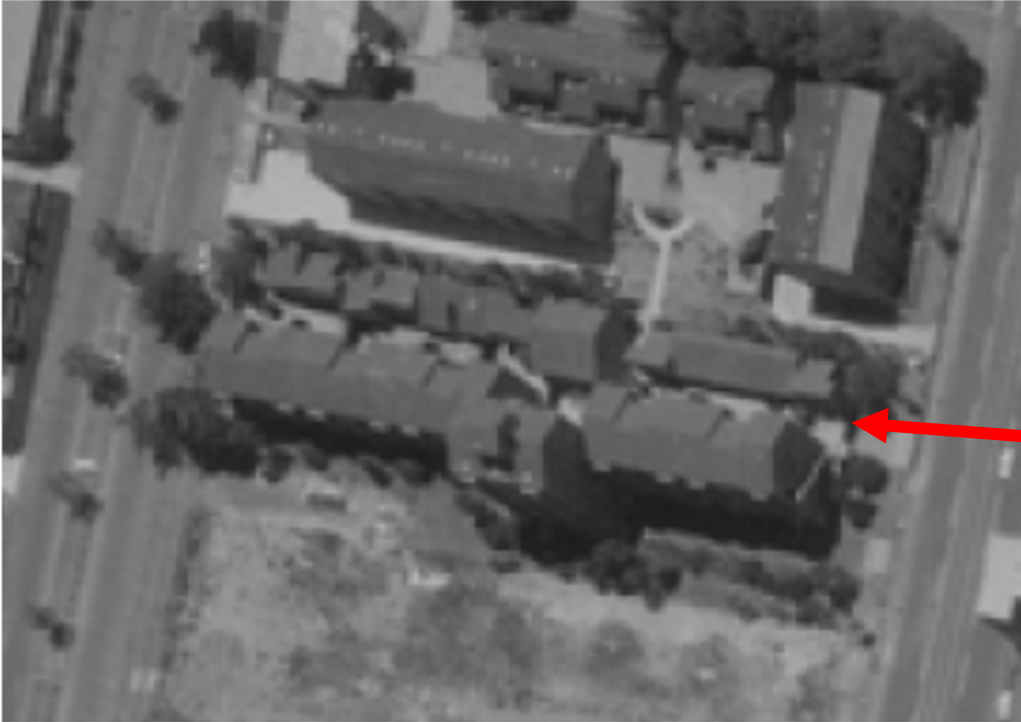
Figure 8 The subject site in 1979 (arrowed) with the undeveloped Lot 2 adjoining to the south (bottom of image); and the developed 'Northern Land' (top of image) Source: Land Victoria Aerial Photography Collection, Central Plan Office, Landata
