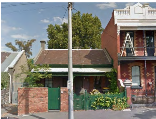
Figure 17 131 Barkly Street, Carlton (HO1) Source: Streetview
