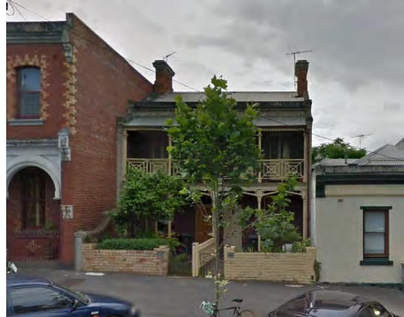
Figure 16 134-6 Barkly Street, Carlton (HO1) Source: Streetview
