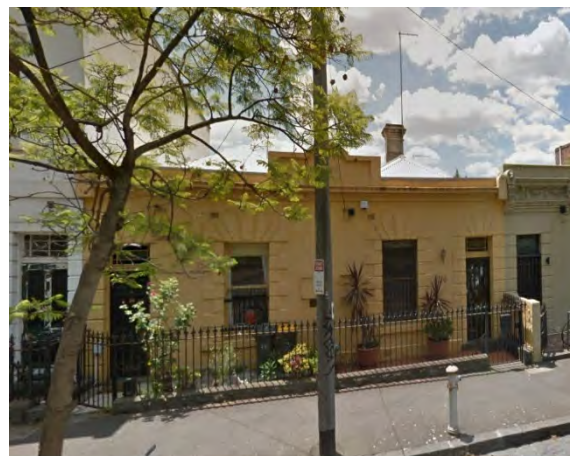
Figure 12 26-8 Barkly Street, Carlton (HO1) Source: Streetview
