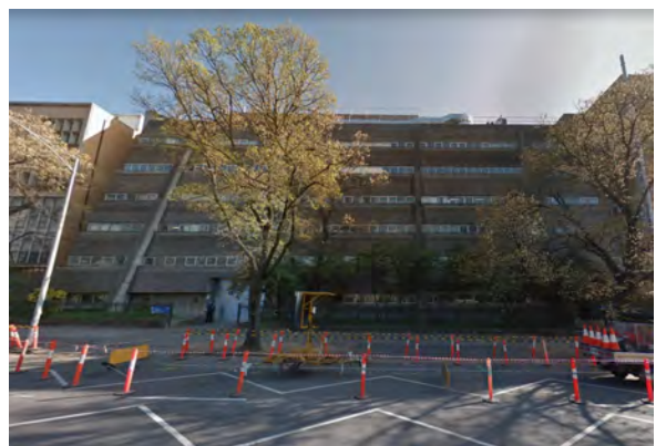
Figure 17 Engineering Faculty, University of Melbourne Source: Google Streetview
