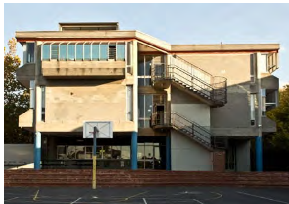
Figure 16 Princes Hill High School, 47 Arnold Street, Princes Hill (1970-73, City of Yarra, HO329) Source: Docomomo
