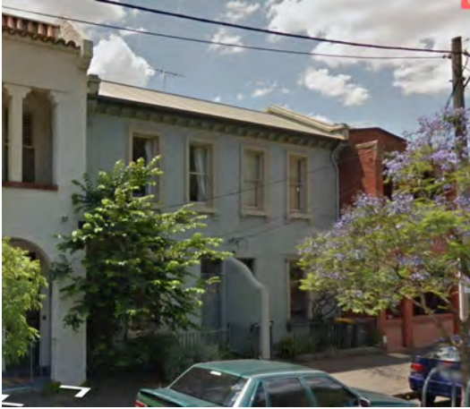
Figure 15 38 Carlton Street, Carlton (HO1) Source: Streetview
