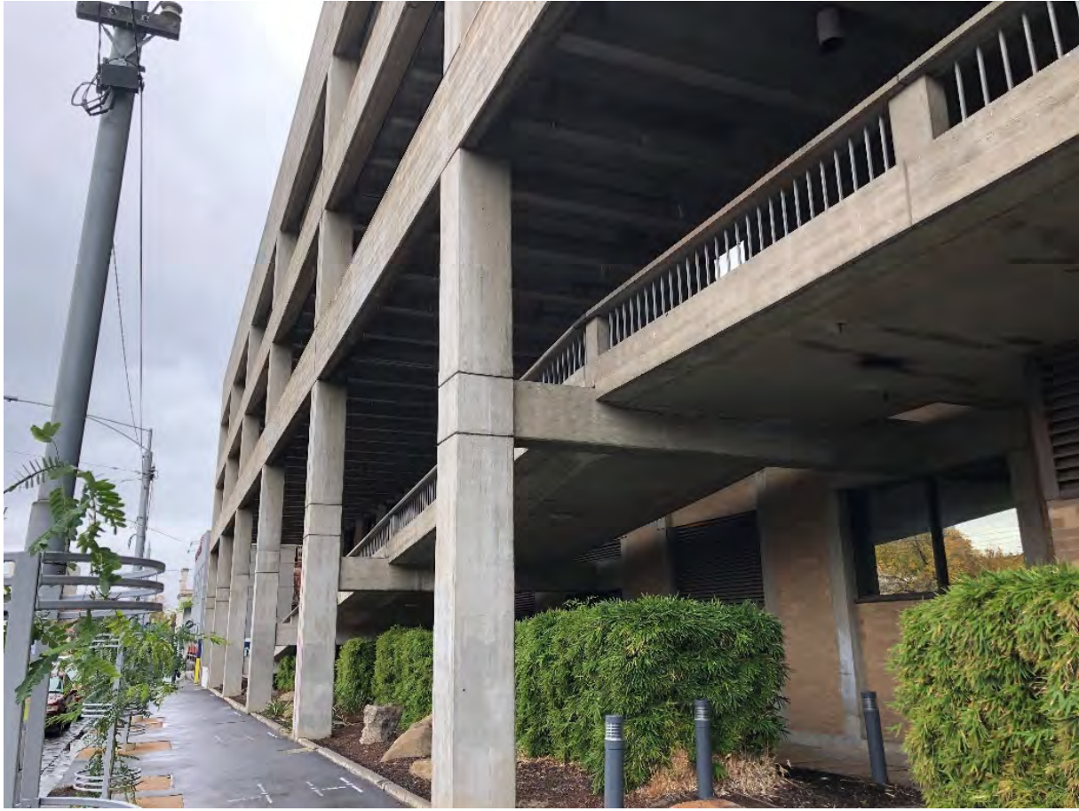
Figure 10 Detail of the concrete ramp, and its underside, which comes up from the east end of the building (in the distance) within the double-height colonnaded loggia Source: Lovell Chen
