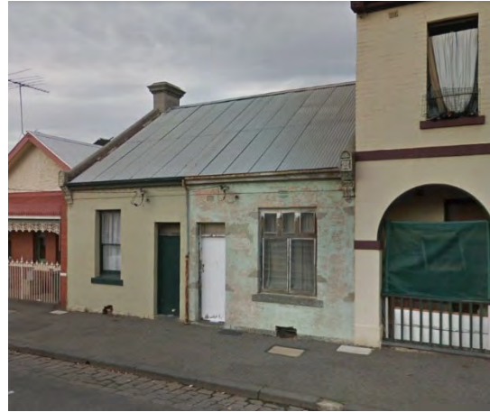
Figure 10 126-8 Station street, Carlton (HO1) Source: Streetview
