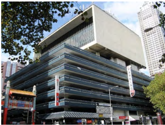
Figure 14 Total carpark, Melbourne, VHR H2329 and HO507 Source: Victorian Heritage Database
