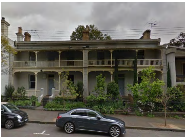
Figure 11 82-4 Carlton Street, Carlton (HO1) Source: Streetview
