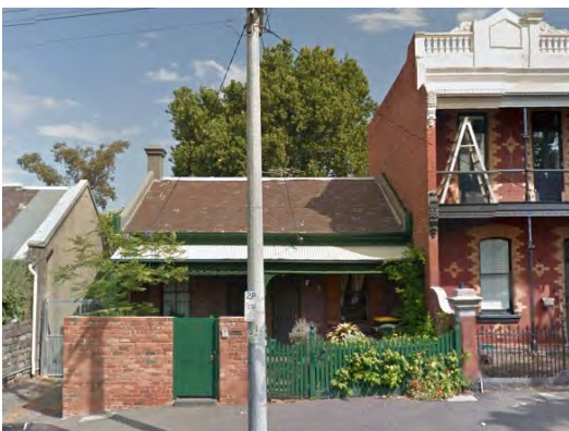
Figure 19 131 Barkly Street, Carlton (HO1) Source: Streetview
