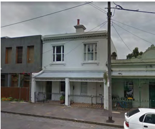
Figure 17 36 Macarthur Place North, Carlton (HO1) Source: Streetview
