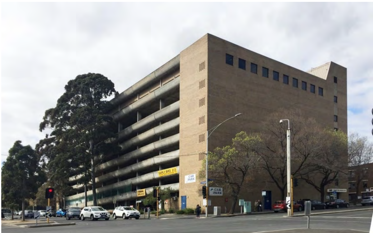
Figure 8 The carpark as viewed from the corner of Grattan and Cardigan streets Source: Lovell Chen
