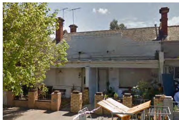
Figure 18 323-234 Faraday Street, Carlton (HO1) Source: Streetview
