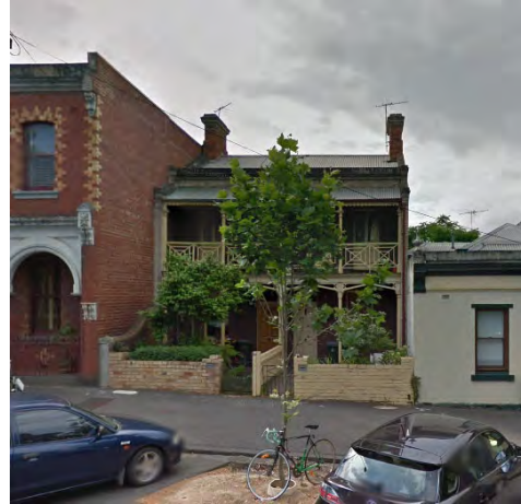
Figure 14 134-6 Barkly Street, Carlton (HO1) Source: Streetview
