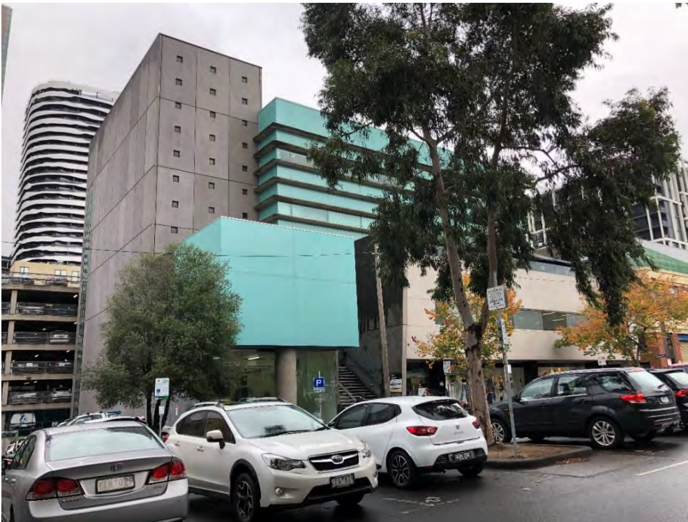
Figure 10 Subject building, viewed from the south; the grey concrete service block is at left, fronted by the southern bay clad in blue-green mosaic tiles Source: Lovell Chen
