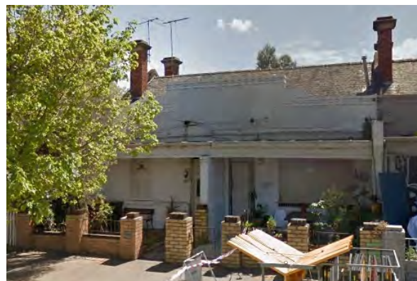
Figure 20 323-234 Faraday Street, Carlton (HO1) Source: Streetview
