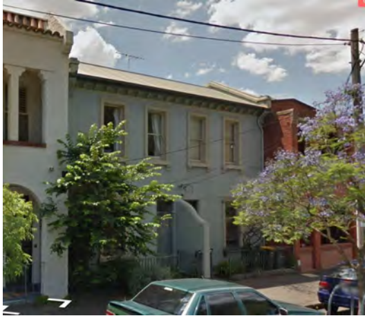
Figure 13 38 Carlton Street, Carlton (HO1) Source: Streetview
