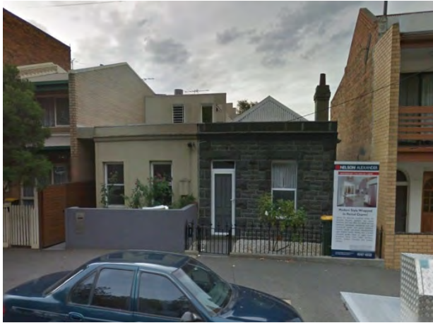
Figure 9 46 Palmerston Street, Carlton (HO1) Source: Streetview
