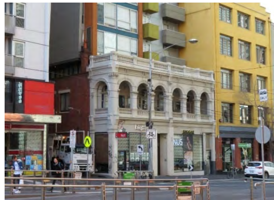
Figure 22 466 Swanston Street, Carlton (HO111) Source: Lovell Chen
