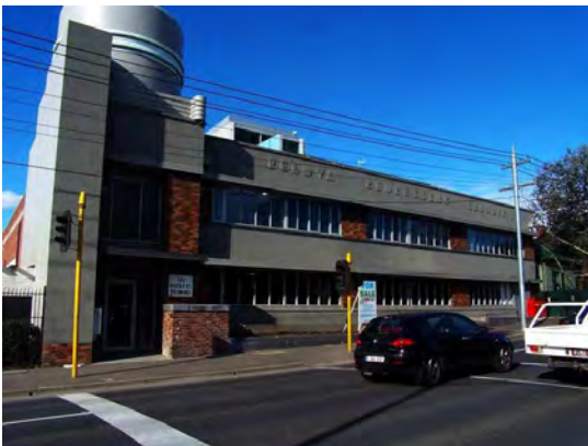
Figure 10 129 Hoddle Street, Richmond (HO391) Source: Victorian Heritage Database
