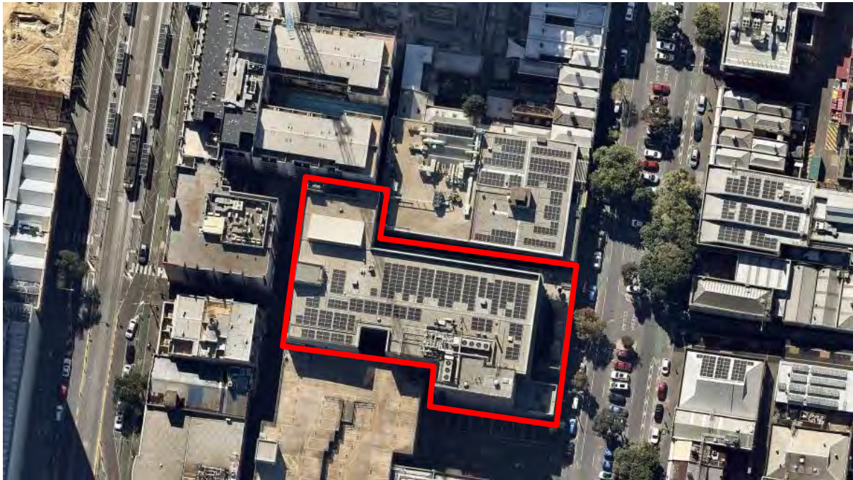
Figure 8 Recent aerial photograph with the subject site indicated Source: Nearmap, April 2019
