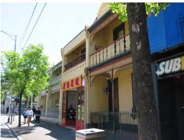
Figure 23 676-82 Swanston Street, Carlton (HO116) Source: Lovell Chen
