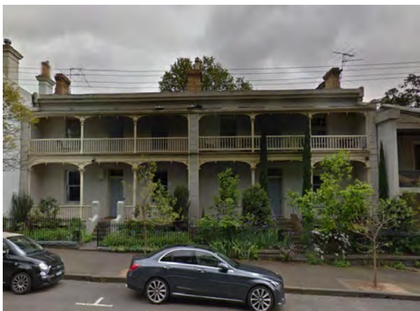
Figure 13 82-4 Carlton Street, Carlton (HO1) Source: Streetview
