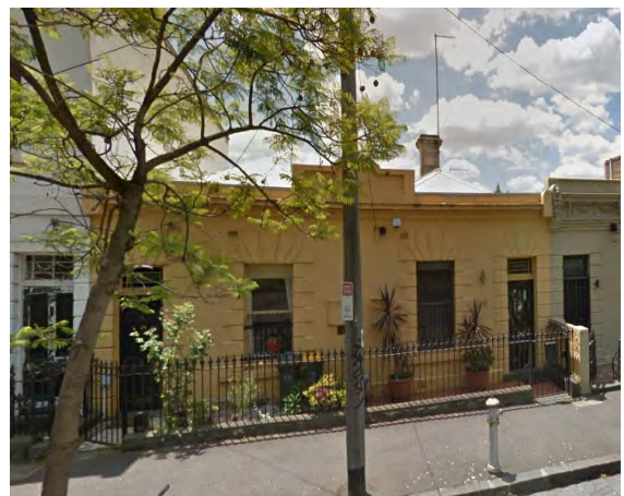
Figure 14 26-8 Barkly Street, Carlton (HO1) Source: Streetview
