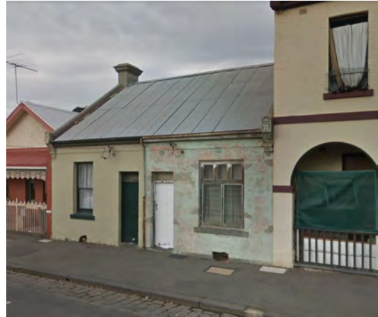
Figure 12 126 Station street, Carlton (HO1) Source: Streetview
