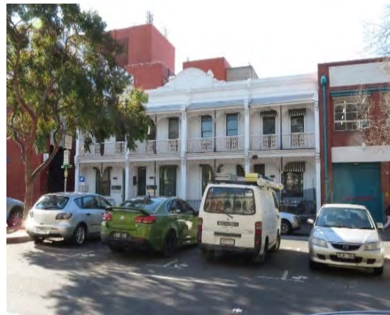
Figure 16 Mary's Terrace, 50-6 Cardigan Street, Carlton (HO36) Source: Lovell Chen
