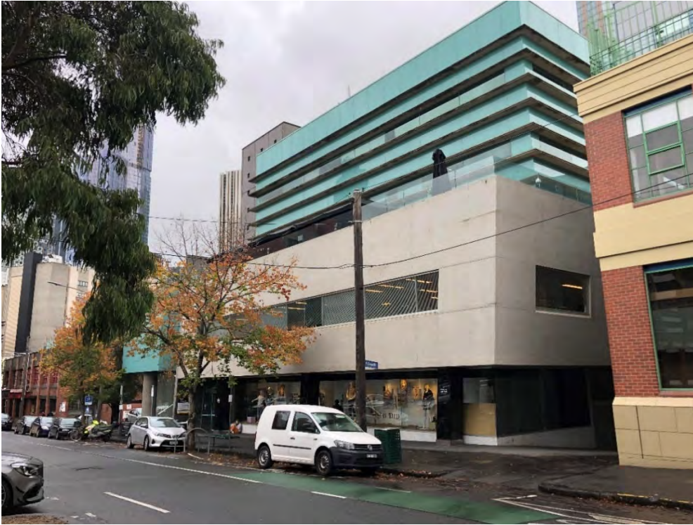
Figure 9 Subject building, viewed from the north; the projecting northern bay at centre is clad in off-white mosaic tiles, with the large volume above clad in blue-green coloured glass Source: Lovell Chen
