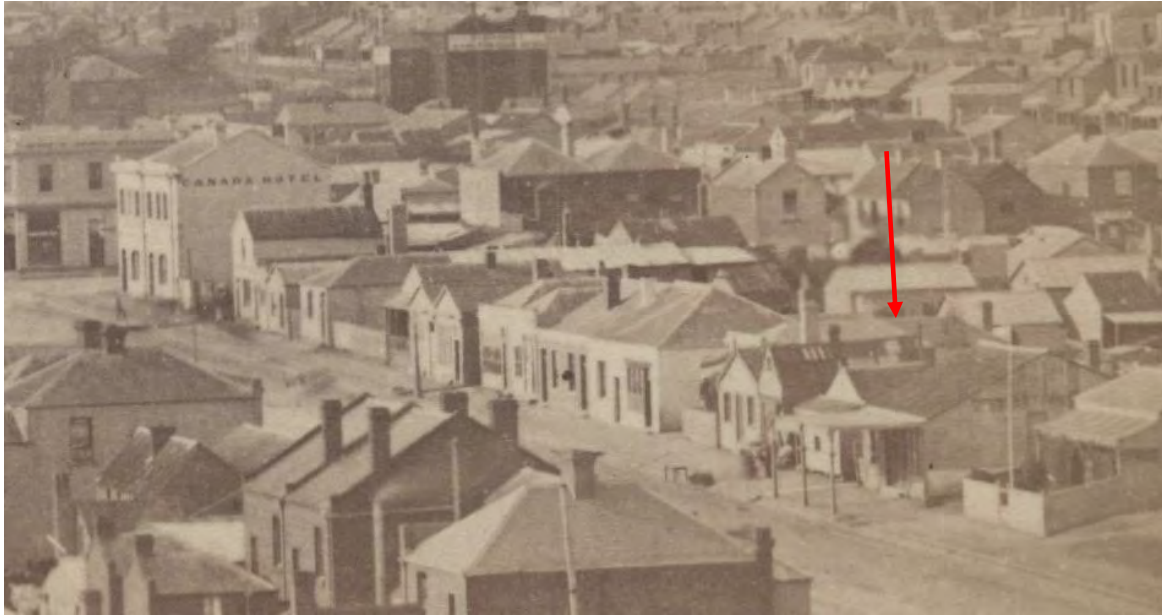
Figure 2 View from Carlton Brewery of east side of Swanston Street between Queensberry and Pelham streets, Carlton, 1870. Approximate location of subject site indicated (prior to construction of the current buildings)
