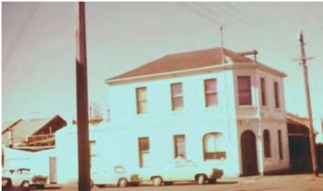
Figure 4 Former Sir John Young Hotel, c. 1974 Source: National Trust, B3393, Victorian Heritage Database
