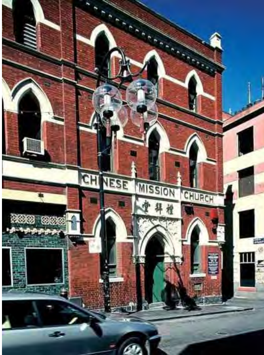
Figure 30 Chinese Mission Church, 119 - 125 Little Bourke Street, Melbourne (1902, HO690 and HO507)
