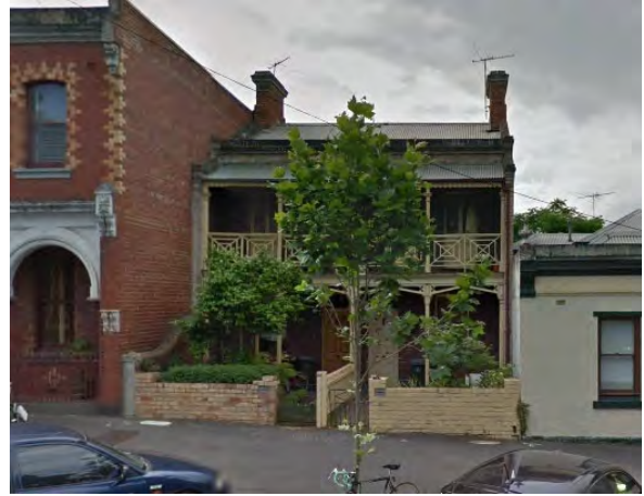
Figure 11 134-6 Barkly Street, Carlton (HO1) Source: Streetview
