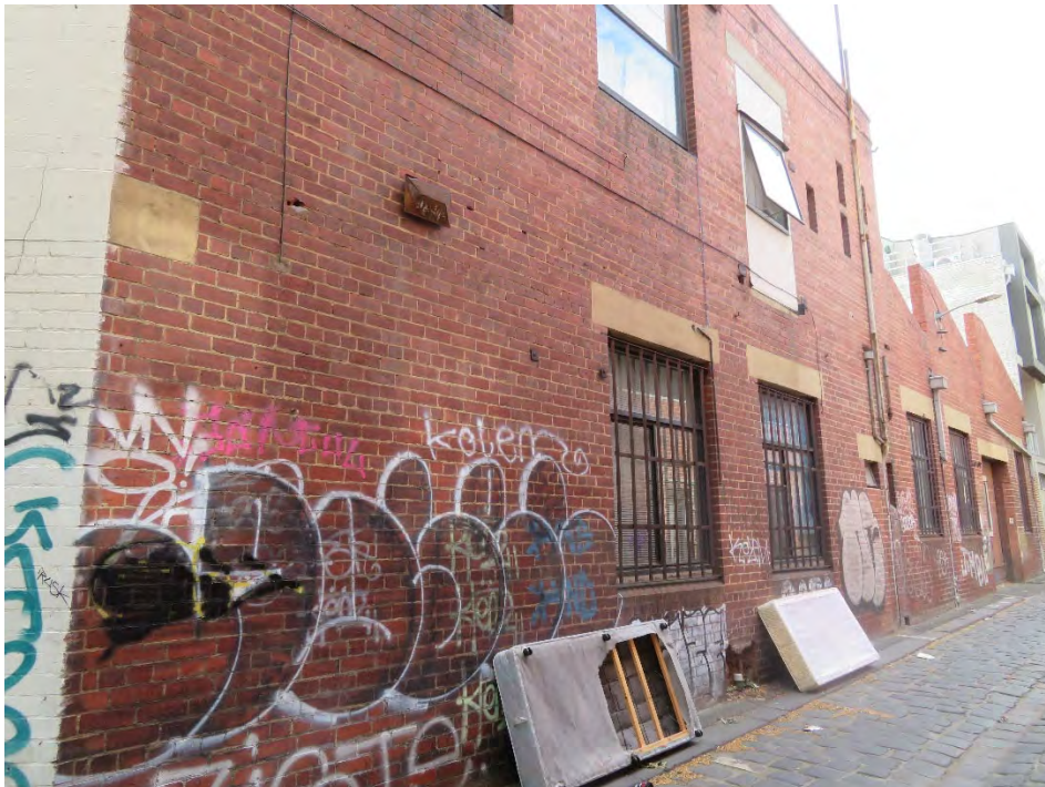
Figure 17 144-146 Queensberry Street, Carlton viewed from Queensberry Lane
