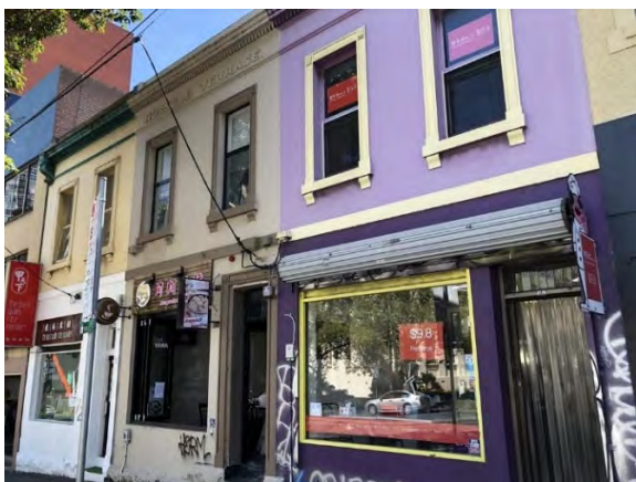
Figure 10 Russell Terrace, 68-72 Victoria Street (HO118) Source: Lovell Chen
