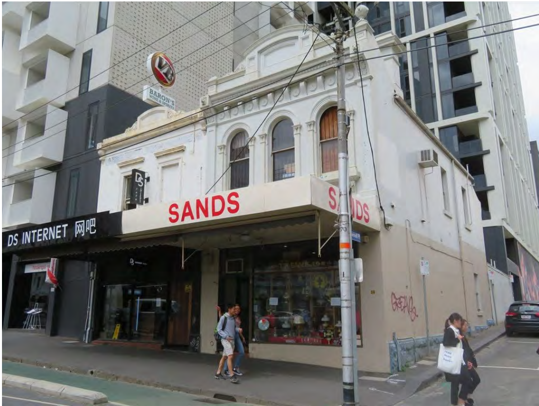
Figure 7 Shops at 508 and 510 –512 Swanston Street, Carlton
