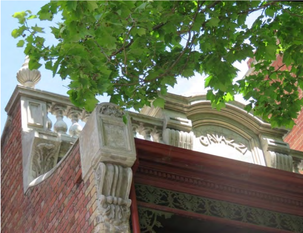
Figure 9 19 Queensberry Street, parapet details
