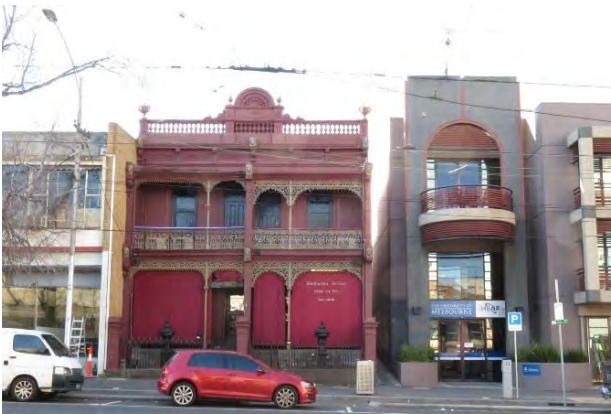
Figure 18 454-6 Swanston Street, Carlton (HO113) Source: Lovell Chen
