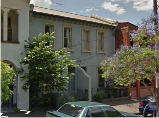
Figure 14 38 Carlton Street, Carlton (HO1) Source: Streetview
