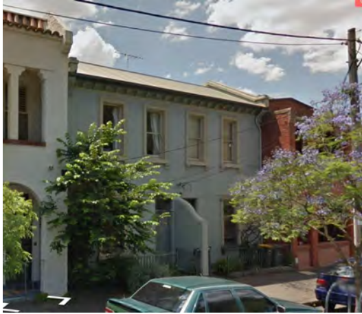
Figure 10 38 Carlton Street, Carlton (HO1) Source: Streetview
