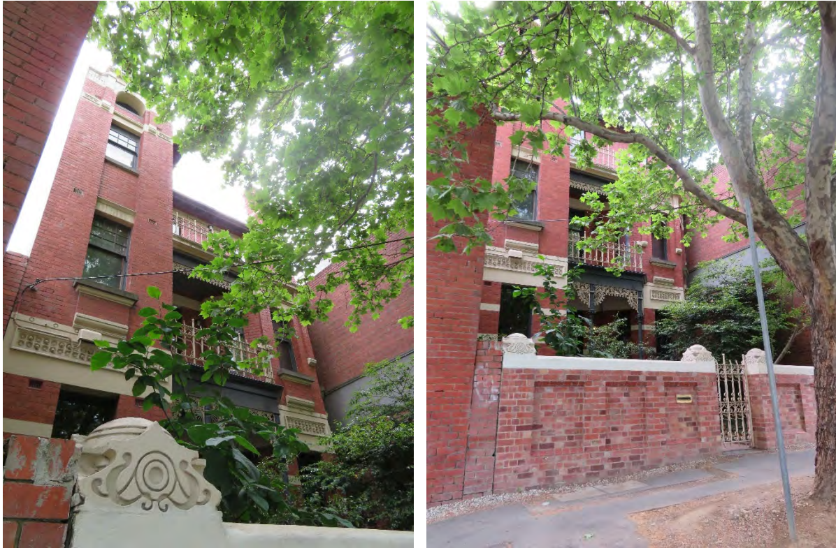
Figure 8 25-7 Rathdowne Street, Carlton; note the central recessed verandah rising up through the building levels
