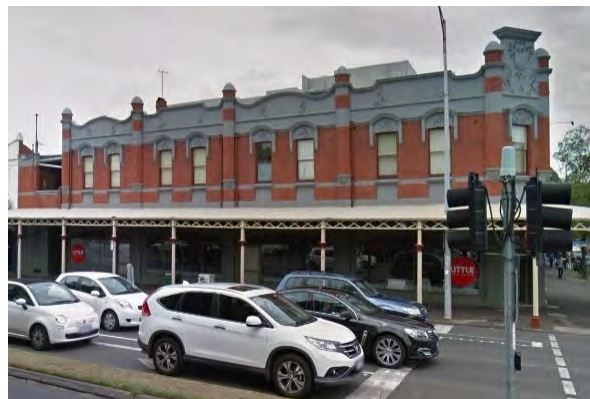
Figure 14 118-120 Elgin Street, Carlton (part HO1) Source: Google Streetview
