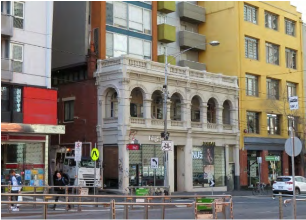
Figure 22 466 Swanston Street, Carlton (HO113) Source: Lovell Chen
