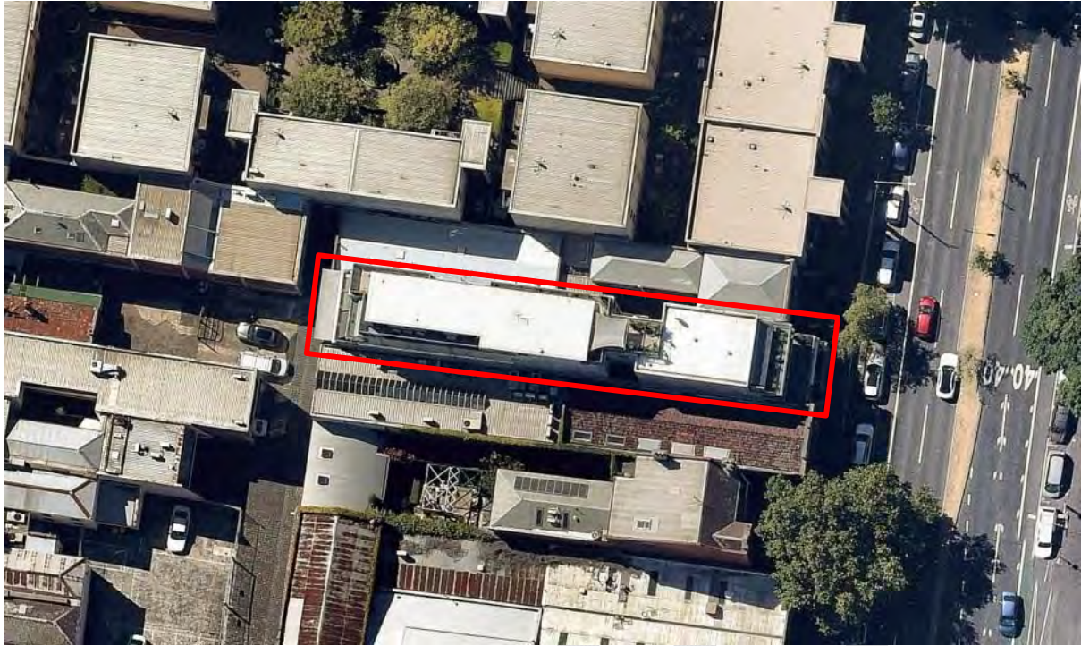
Figure 6 Recent aerial photograph of the subject site Nearmap, February 2019
