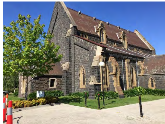
Figure 12 South Yarra Presbyterian Church, 621 Punt Road, South Yarra (HO6) Source: Lovell Chen
