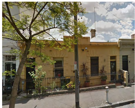
Figure 9 26-8 Barkly Street, Carlton (HO1) Source: Streetview
