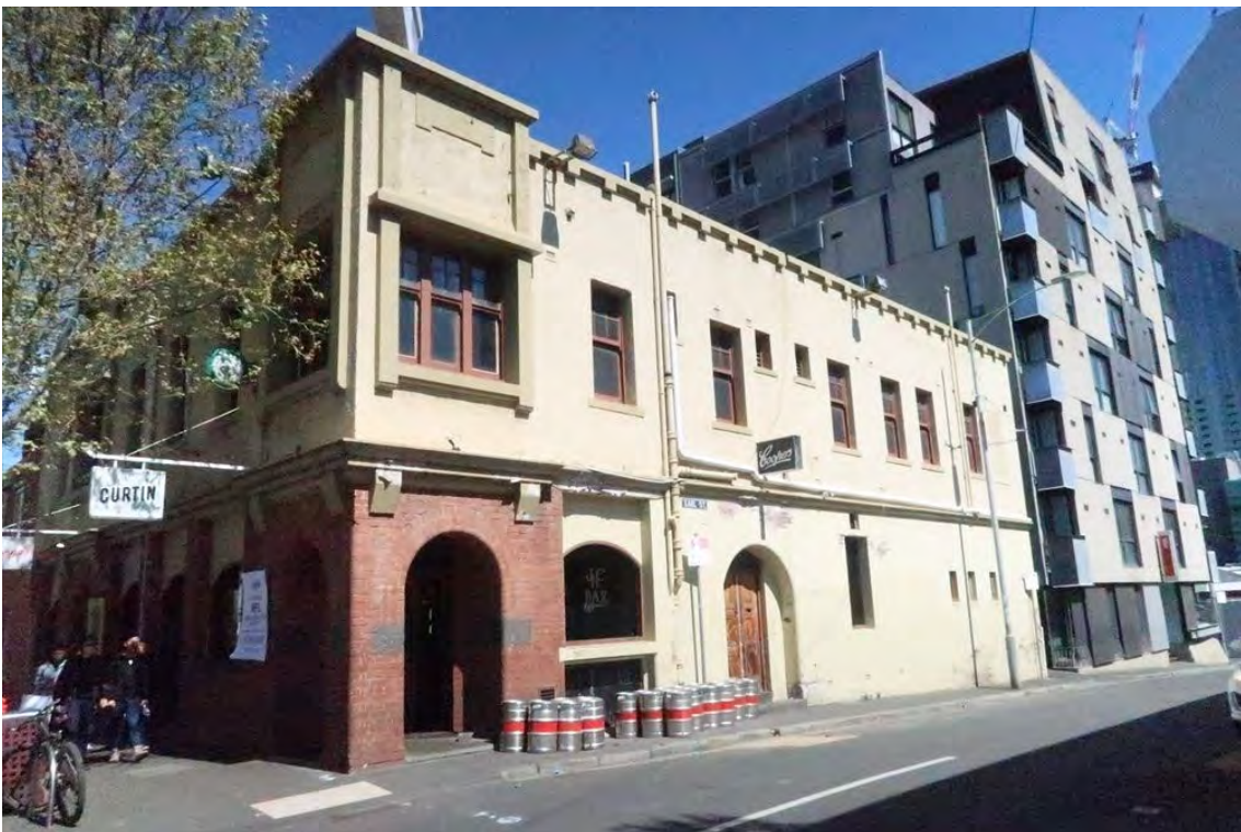
Figure 14 John Curtin Hotel, viewed from the intersection of Earl and Lygon streets
