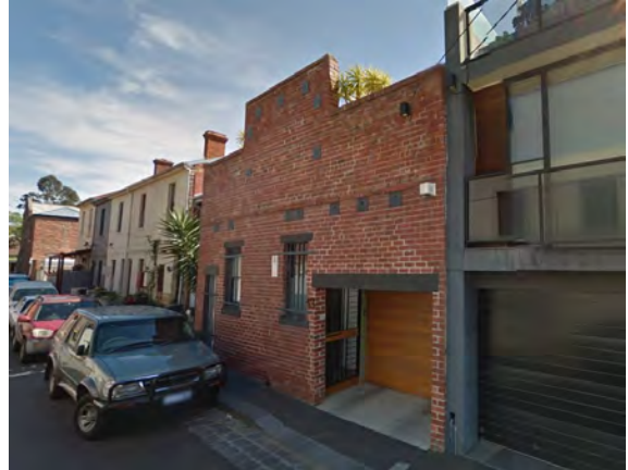
Figure 9 13-23 David Street, Carlton (HO1) Source: Streetview
