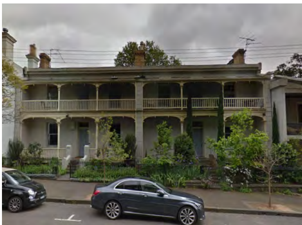
Figure 8 82-4 Carlton Street, Carlton (HO1) Source: Streetview
