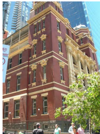
Figure 15 Former Queen Victoria Hospital Tower (H0956) Source: Victorian Heritage Database
