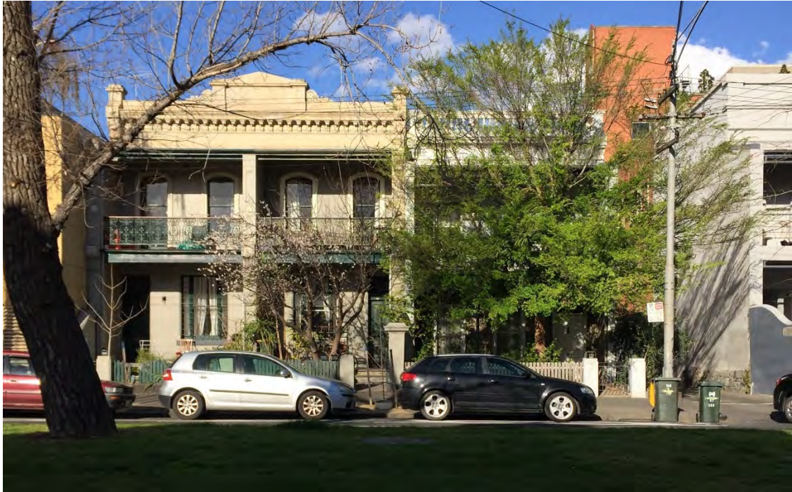
Figure 10 112-114 Drummond Street on the left and 110 Drummond Street on the right concealed by the tree
