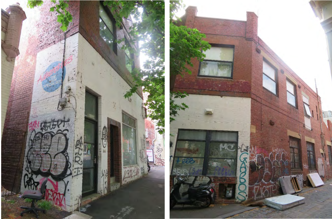
Figure 16 144-146 Queensberry Street, Carlton viewed from the south-west (at left) and from the south-east (at right)
