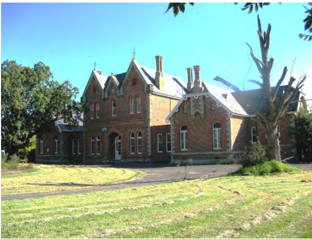
Figure 14 Former Bairnsdale Hospital (H2310) Source: Victorian Heritage Database
