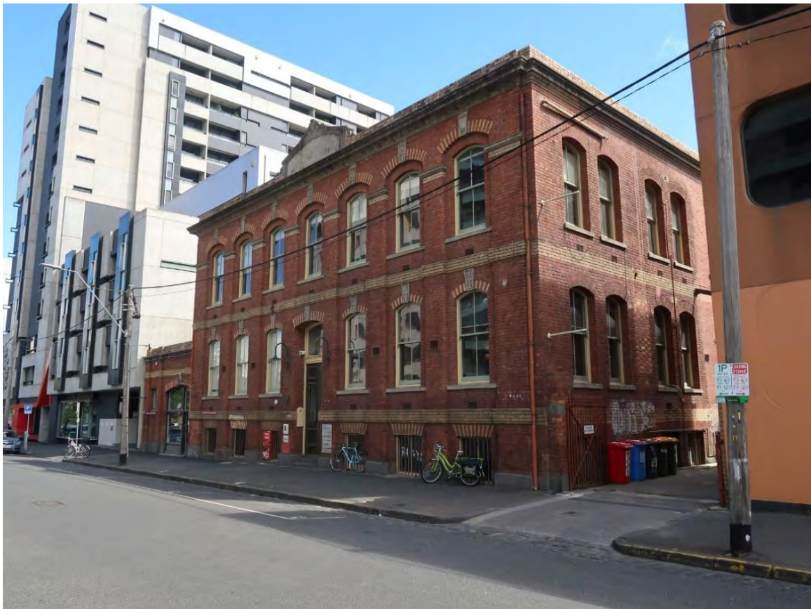
Figure 12 96-106 Pelham Street, Carlton
