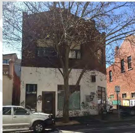
Figure 11 144-146 Queensberry Street, Carlton (HO807) Source: Lovell Chen
