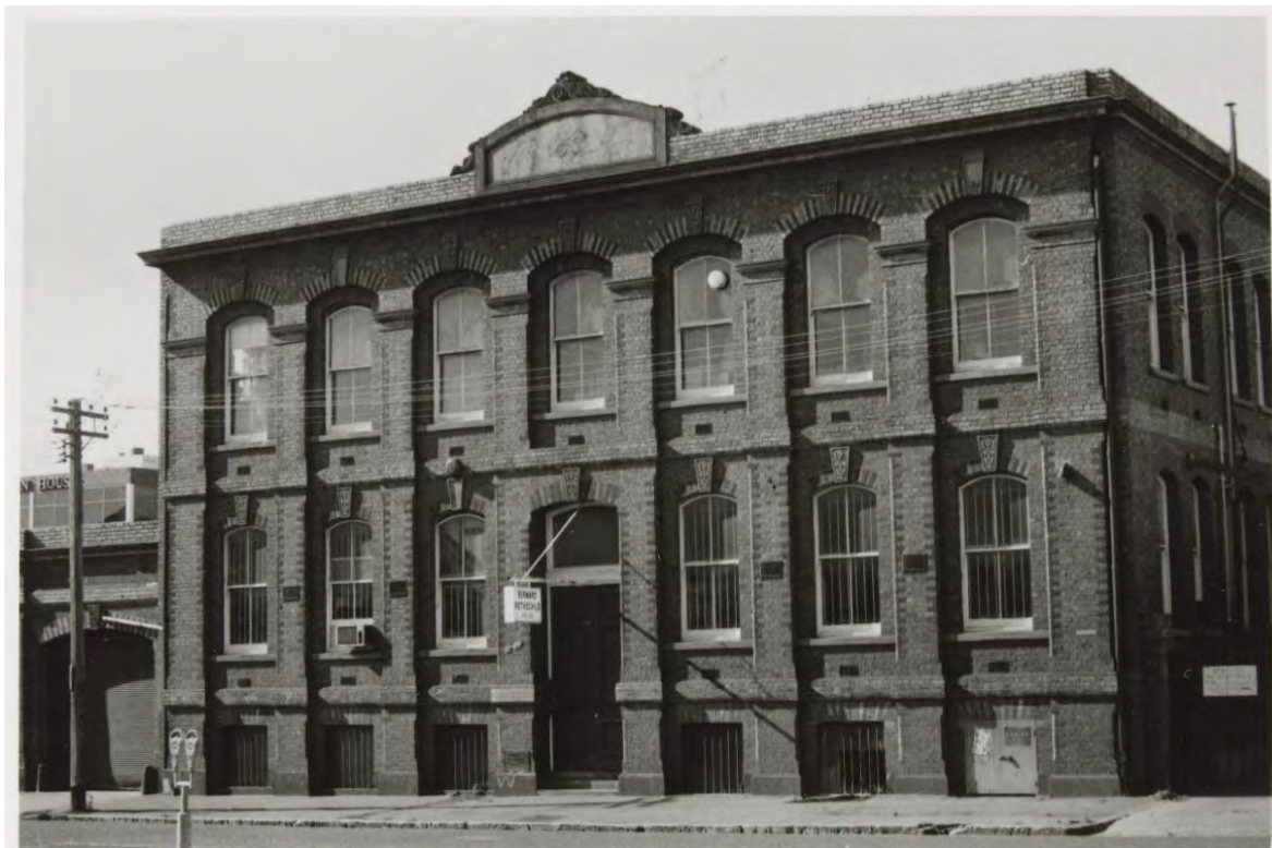
Figure 10 Subject building, 1982; note the carriage gate at left Source: J T Collins collection, H94.200/227, State Library of Victoria
