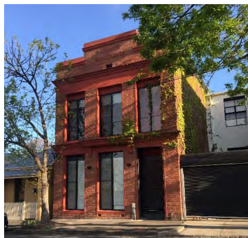
Figure 13 49 Owen Street, Carlton (HO1) Source: Lovell Chen
