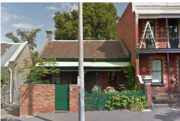
Figure 18 131 Barkly Street, Carlton (HO1) Source: Streetview
