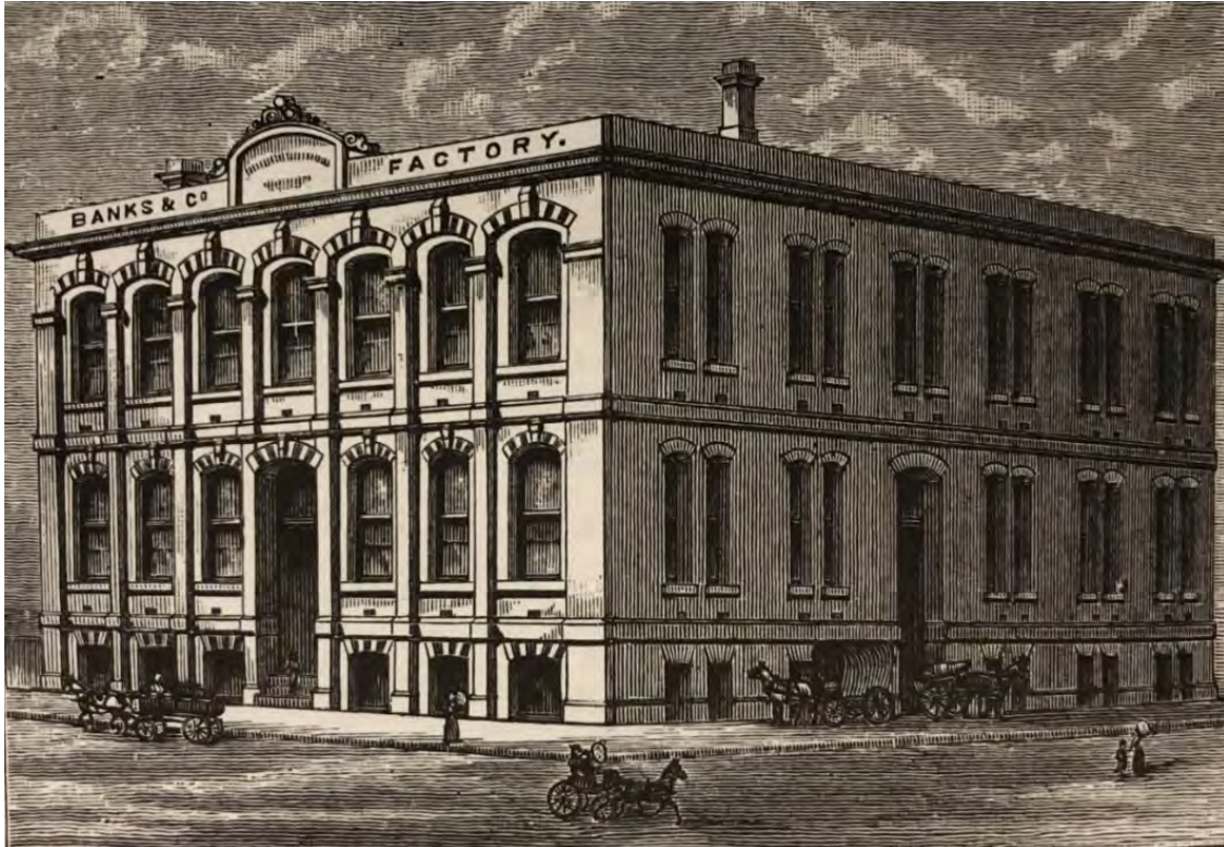
Figure 4 Banks & Co's factory, Pelham Street, 1888 Source: Victoria and its Metropolis, Past and Present , Vol. IIB, p. 592, facsimile edition, Today's Heritage, 1977.
