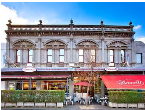
Figure 11 Shops at 198-204 Faraday Street, Carlton, Norman Hitchcock architect, 1886 (HO1) Source: Pinterest
