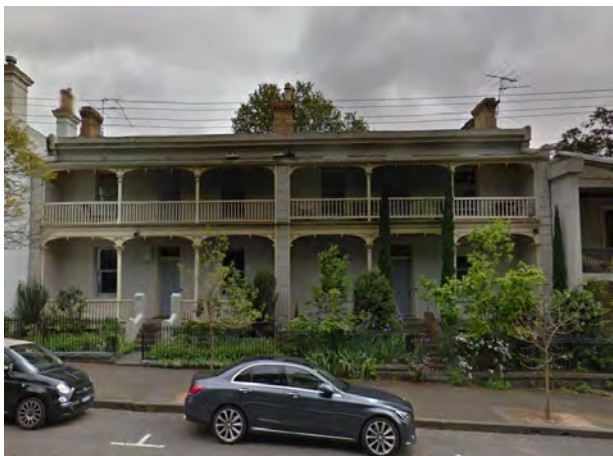
Figure 12 82-4 Carlton Street, Carlton (HO1) Source: Streetview
