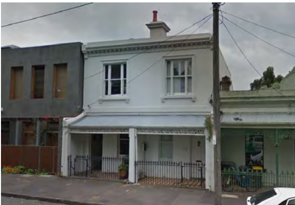
Figure 16 36 Macarthur Place North, Carlton (HO1) Source: Streetview
