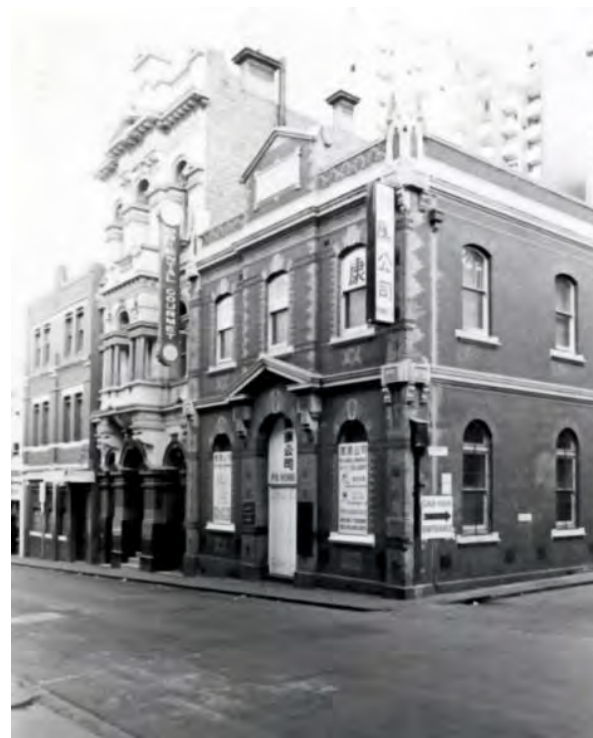
Figure 29 Church of England Mission Hall, 108-110 Little Bourke Street, Melbourne (1884, HO688 and HO507) Source: Victorian Heritage Database
