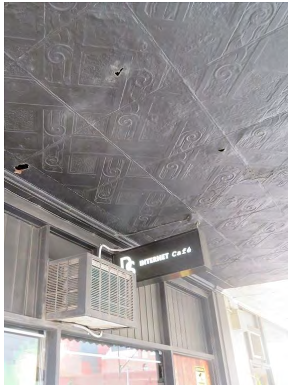
Figure 8 Parapet ornament at no. 508 (at left); pressed metal verandah soffit (at right)
