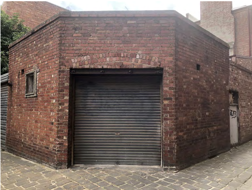
Figure 10 The stable to the rear of 19 Queensberry Street
