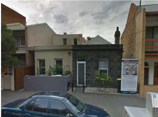
Figure 6 46 Palmerston Street, Carlton (HO1) Source: Streetview
