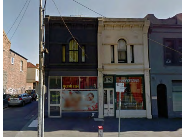
Figure 12 82-84 Elgin Street, Carlton (HO1) Source: Google Streetview
