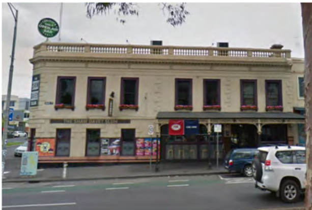
Figure 19 Shaw Davey Slum Hotel, 171-5 Elgin Street, Carlton (HO1) Source: Streetview
