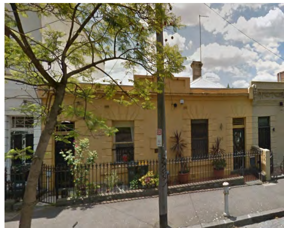
Figure 13 26-8 Barkly Street, Carlton (HO1) Source: Streetview
