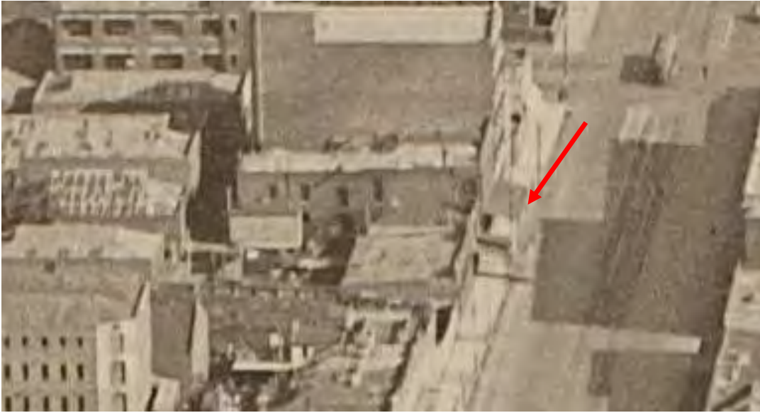
Figure 7 1927 Airspy image with original or early verandah indicated Source: SLV, accession no. H2501
