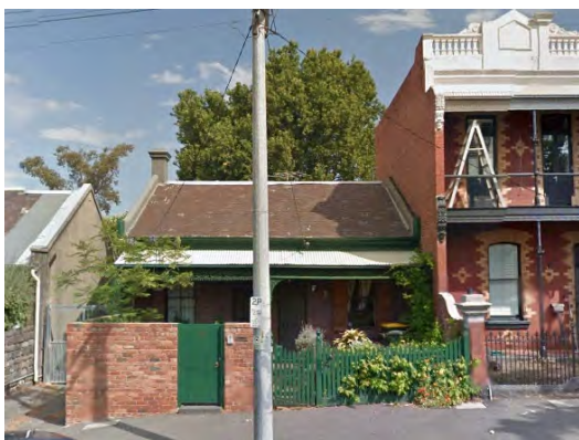
Figure 14 131 Barkly Street, Carlton (HO1) Source: Streetview
