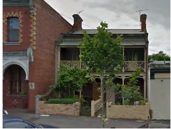
Figure 15 134-6 Barkly Street, Carlton (HO1) Source: Streetview
