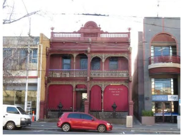
Figure 21 454-6 Swanston Street, Carlton (HO36) Source: Lovell Chen
