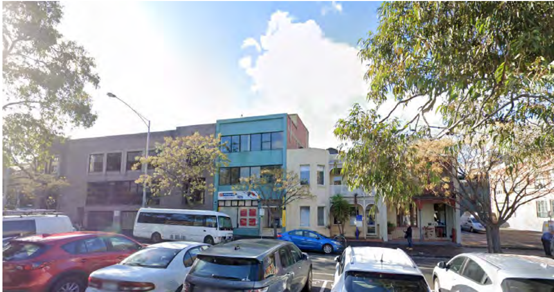
Figure 4: 174-176 (centre-left) and 172 (centre-right) Bouverie Street, Carlton
