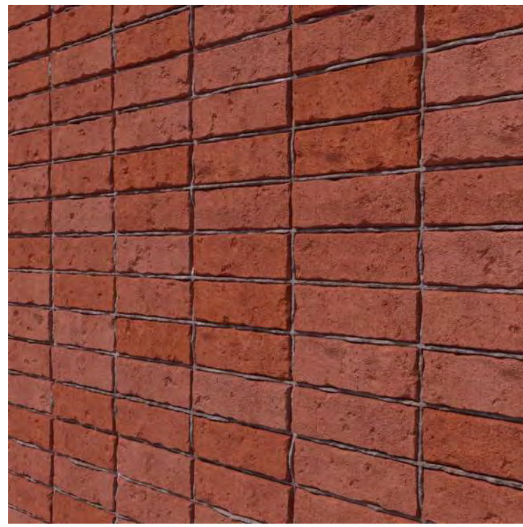
EF-01A RED BRICK 01 - STACK BOND REFERENCE IMAGE
