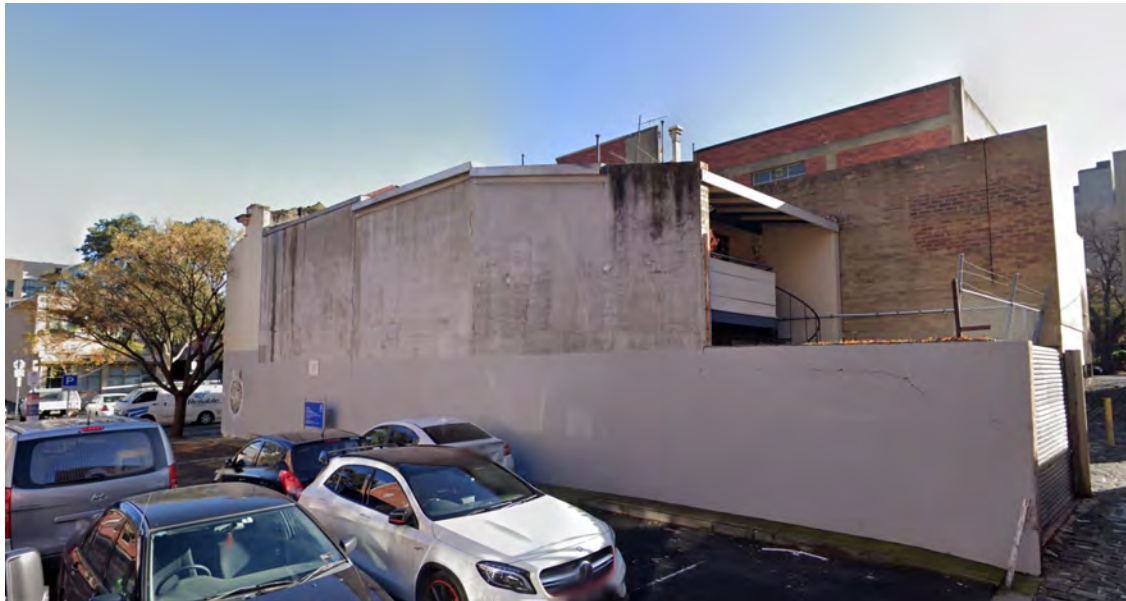
Figure 6: Rear of building at 166-170 Bouverie Street viewed from Church Street
