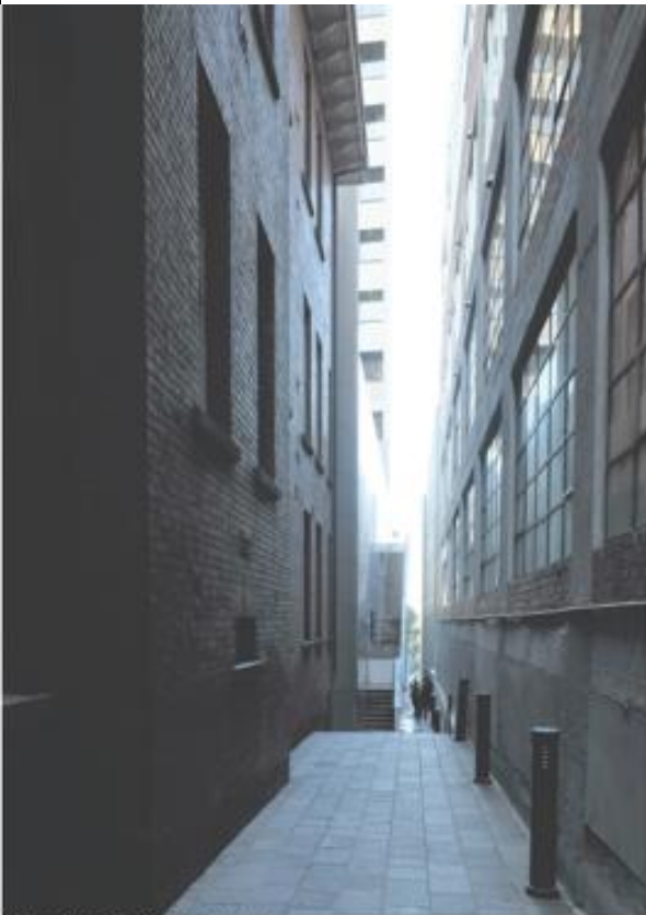
Existing Condition Western Laneway
