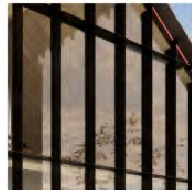
MT01 - STEEL WINDOW FRAME & SHROUD
