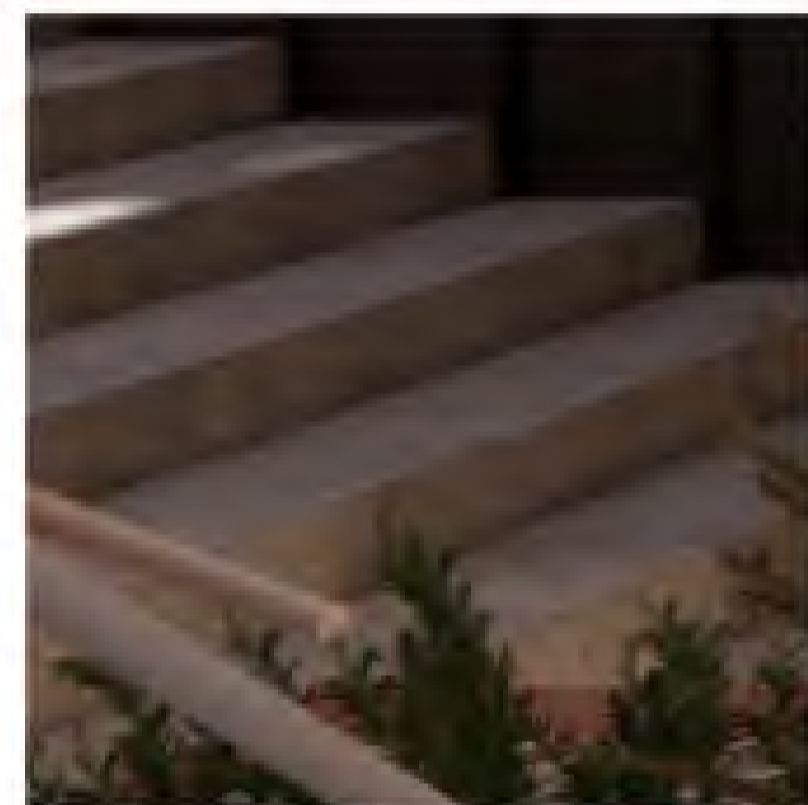
CON01 - CONCRETE COLUMNS AND STEPS
