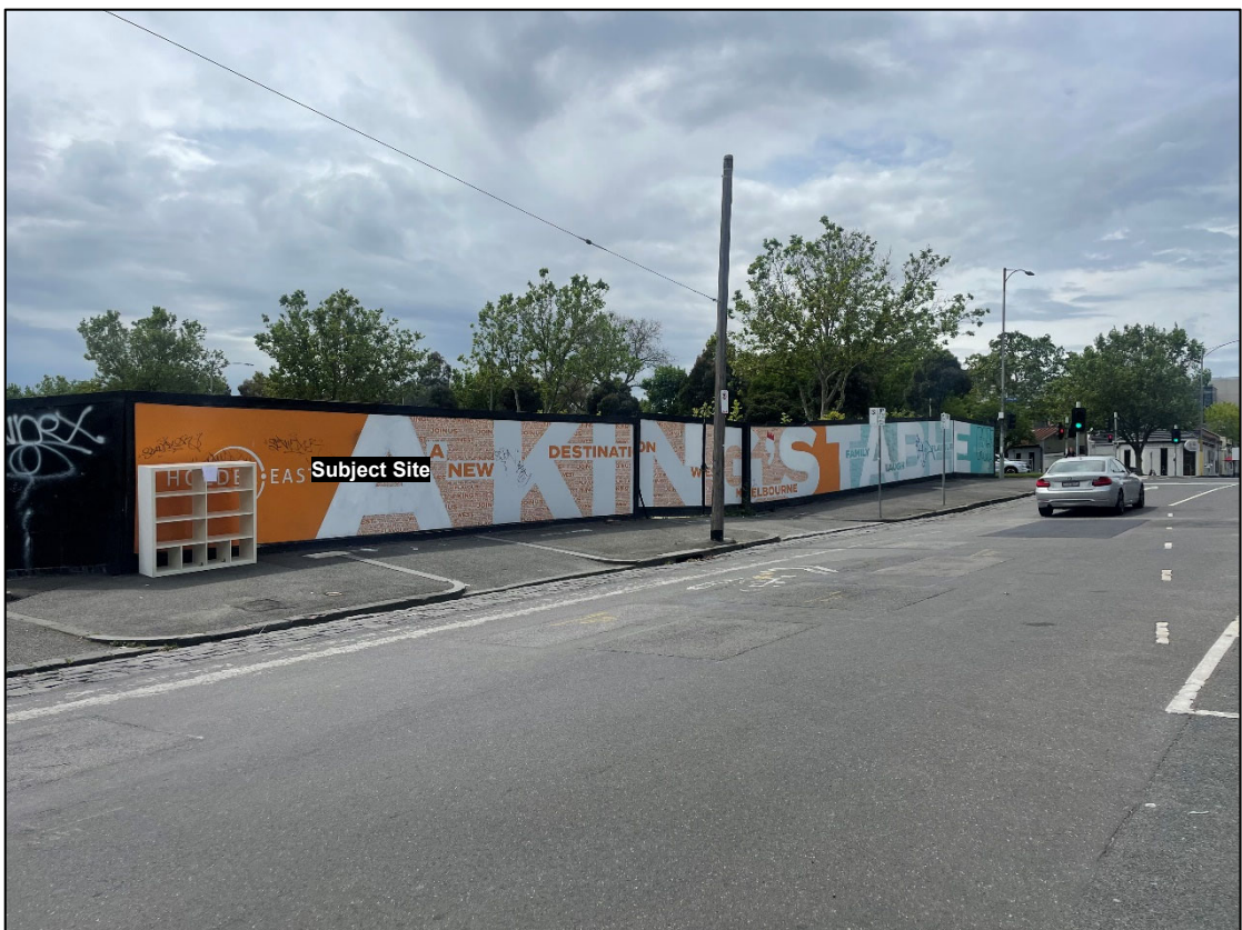
Figure 3 - Subject site as viewed from Rosslyn Street
