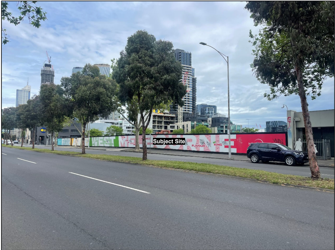
Figure 2 - Subject site as viewed from King Street
