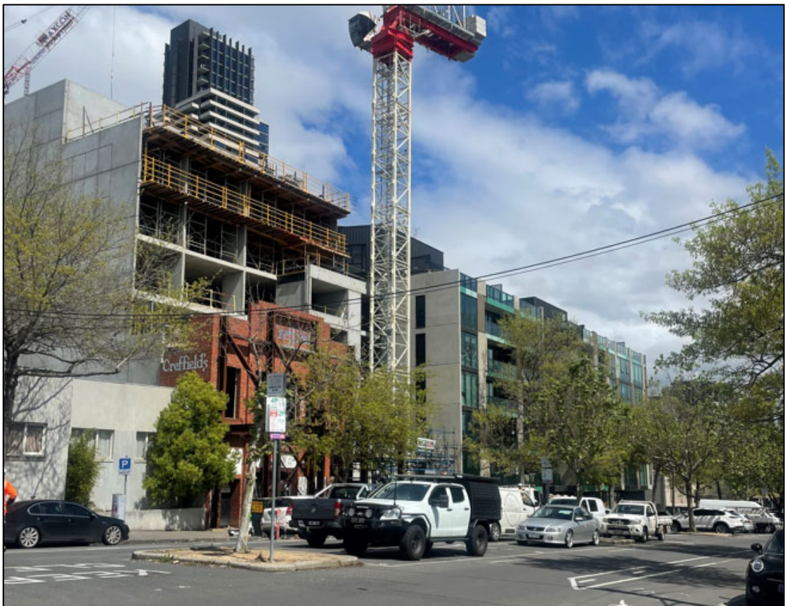
Figure 7 - Built form character along Rosslyn Street
