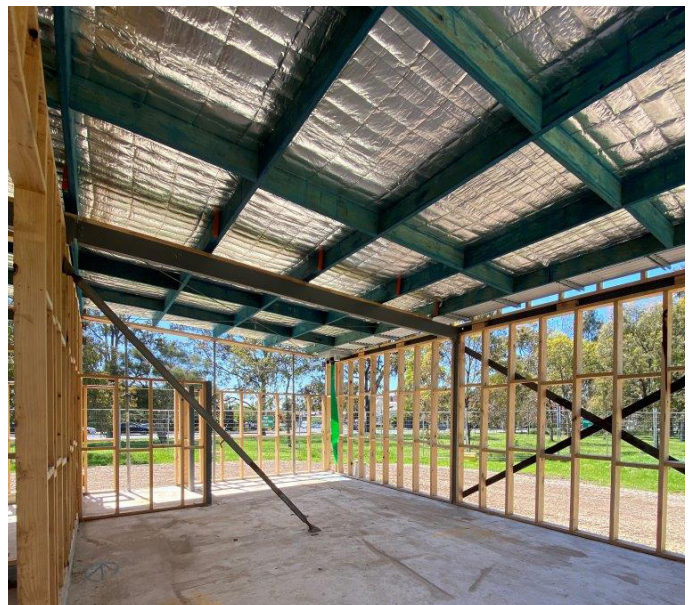
The roof of the new pavilion has been installed
