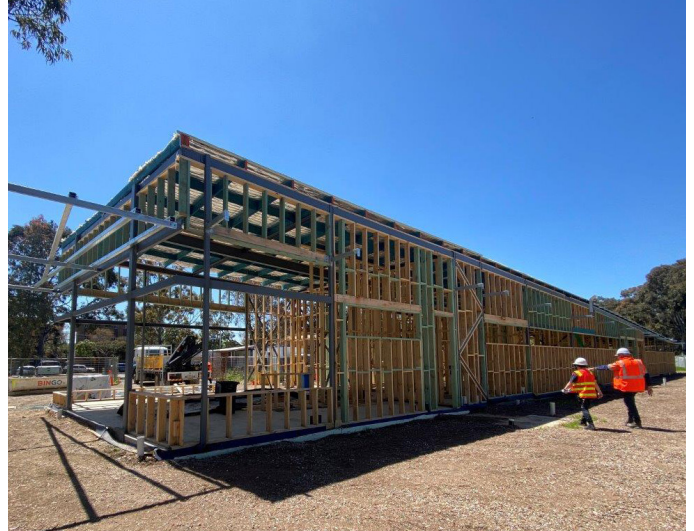
The new building is taking shape
