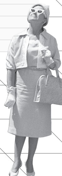
Building Works Outside Melbourne Town Hall (detail) c1961 B & W photograph handprinted from original 2 1/4" negative City of Melbourne Art + Heritage Collection
