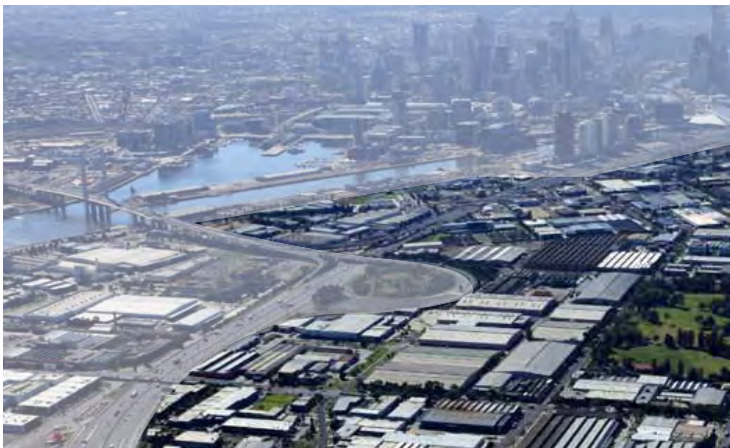
Figure 4: Aerial photograph of the Fishermans Bend Urban Renewal Area today looking towards Docklands and the Hoddle Grid
