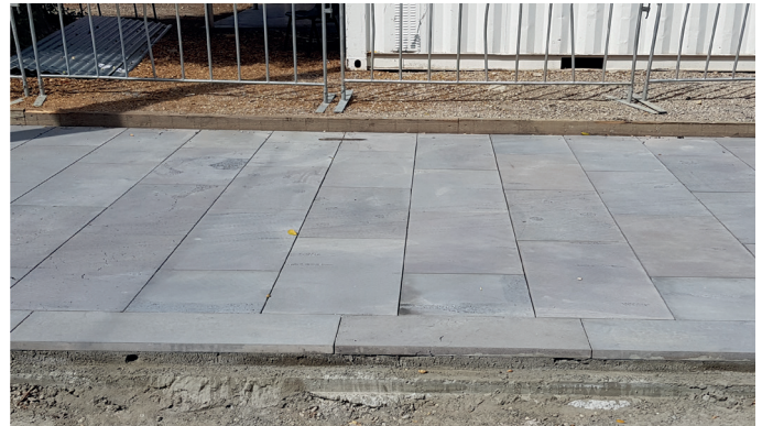
Bluestone pavement currently under construction on Southbank Boulevard
