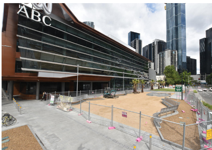
The Civic Space to the front of the ABC nearing completion
